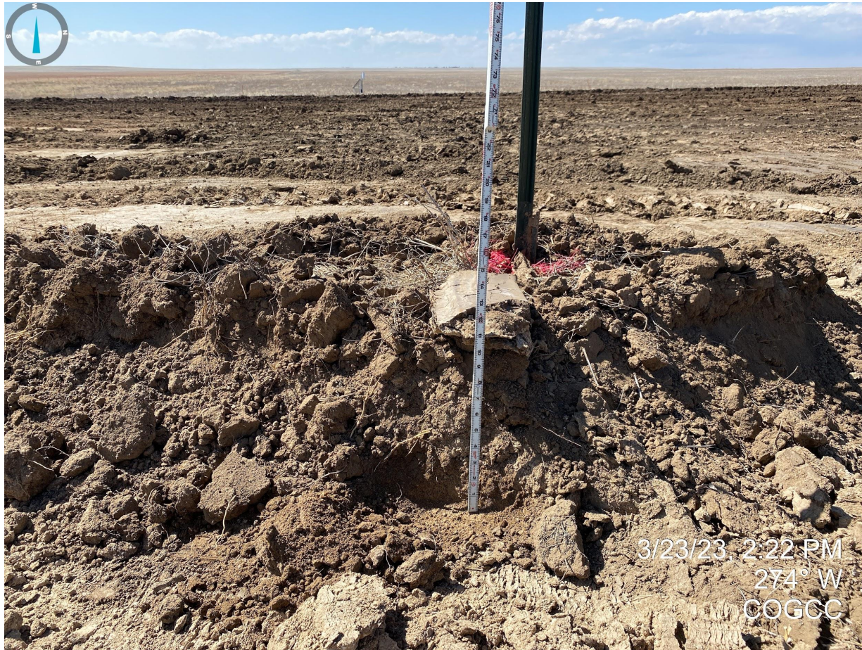
Photo 10. Facing west from the proposed well location; photo illustrates topsoil salvage with rule for scale.
