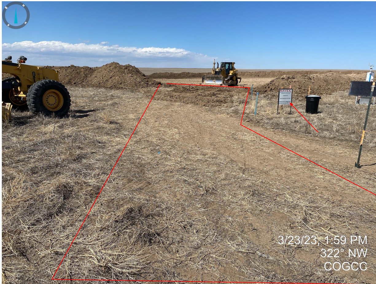
Photo 3. Facing northwest at the construction pad entrance. Photo illustrates that the approach to the pad, and the access road (both outlined in red), have not been salvaged for topsoil and will be required Per Rule 1002.b. Red arrow illustrates location signage that needs to be moved to the entrance for the access road.
