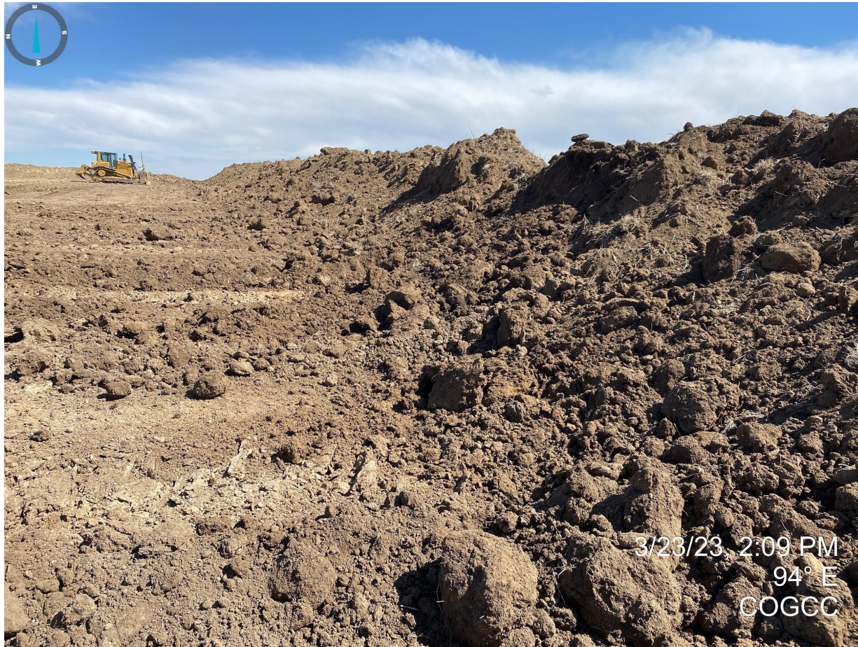
Photo 9. Facing east at the southern topsoil stockpile. Appears the topsoil has been segregated and stockpiled and will need to be stabilized from wind and water erosion. Construction was still on going during this inspection; a follow-up inspection will be conducted to document the topsoil stockpiles for Rule 1002.c compliance.
