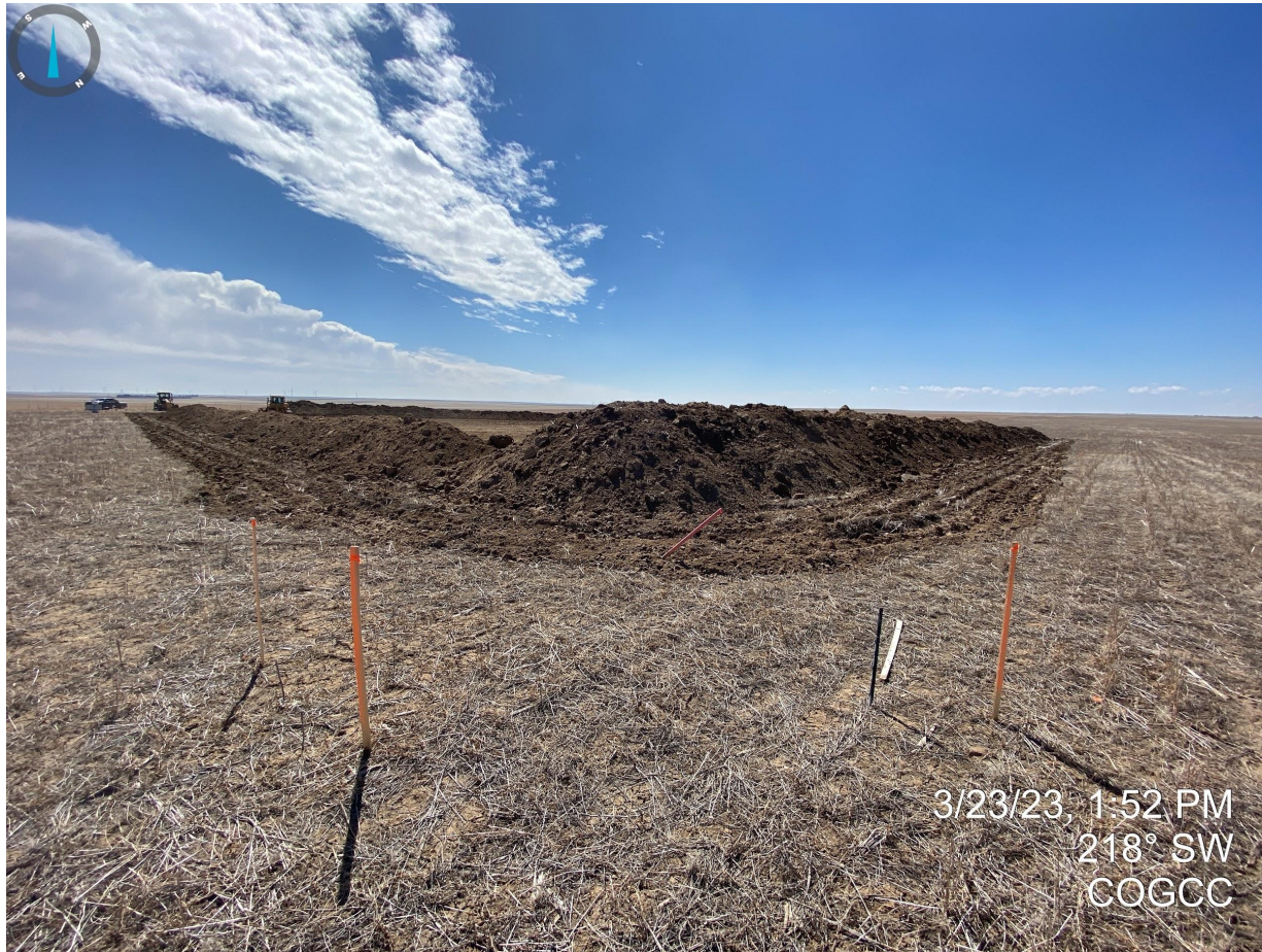
Photo 6. Facing southwest from the northeast corner of the construction. It appears temporary BMPs (surface roughening) have been installed during the initial site construction. On-site contractor advised that straw wattles would be installed at a later date. Some BMPs are still in-process (sediment traps, etc). More permanent stormwater BMPs should be selected after pad construction is completed. Topsoil stockpiles also pictured on the interior perimeter of the disturbance area.
