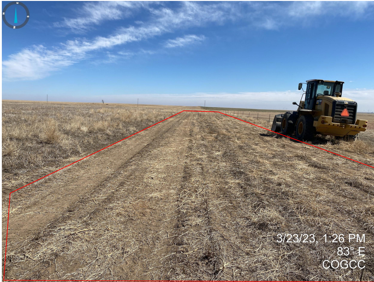
Photo 4. Facing east along access road. Topsoil from the access road has not been salvaged at the time of this inspection.
