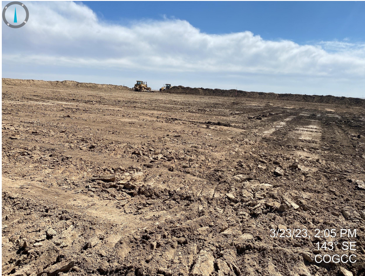
Photo 11. Facing southeast from the northern portion of the location. It appears that topsoil has been salvaged from the location in accordance with Rule 1002.b.
