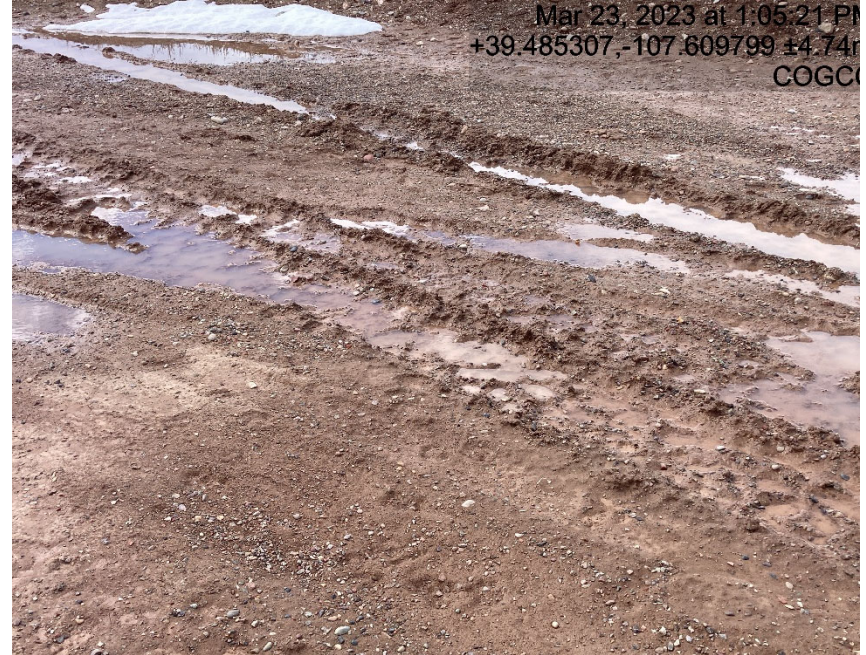
Lack of stabilization/compaction
