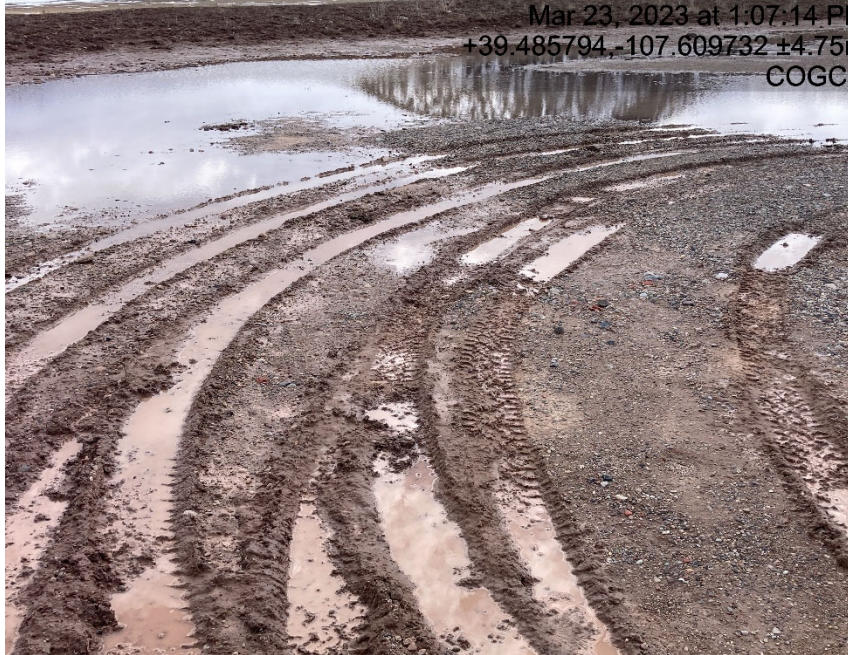
Lack of stabilization/compaction
