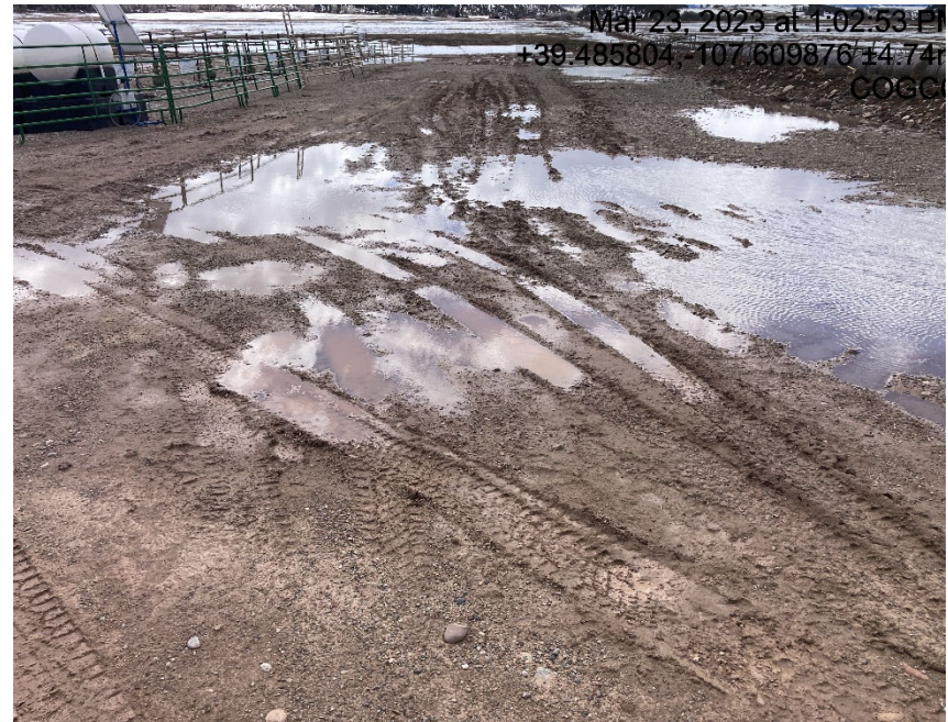
Lack of stabilization/compaction
