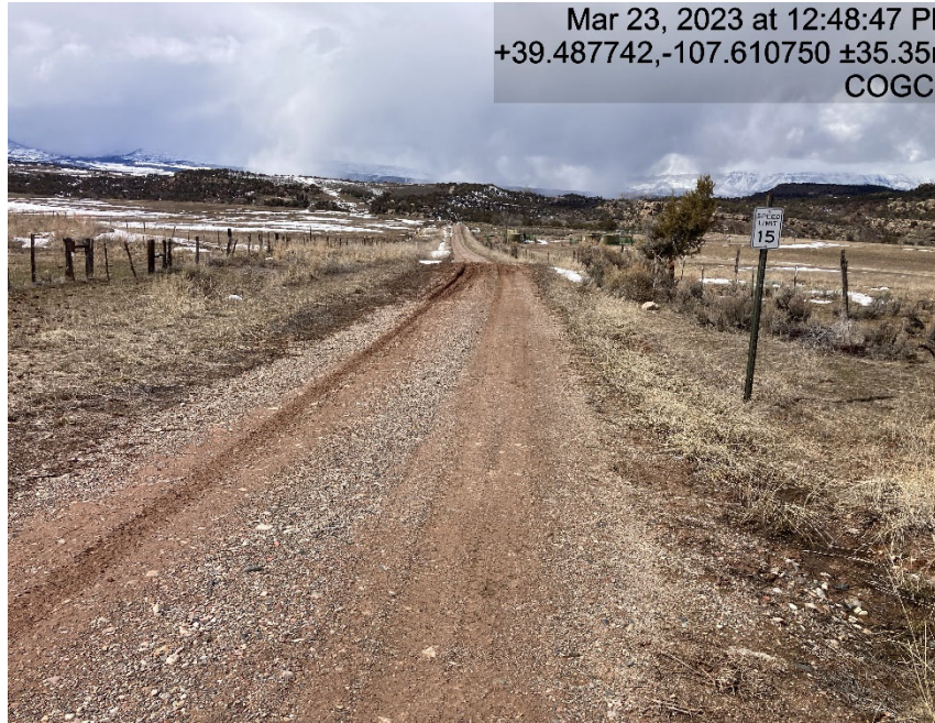
Access road show lack of stabilization
