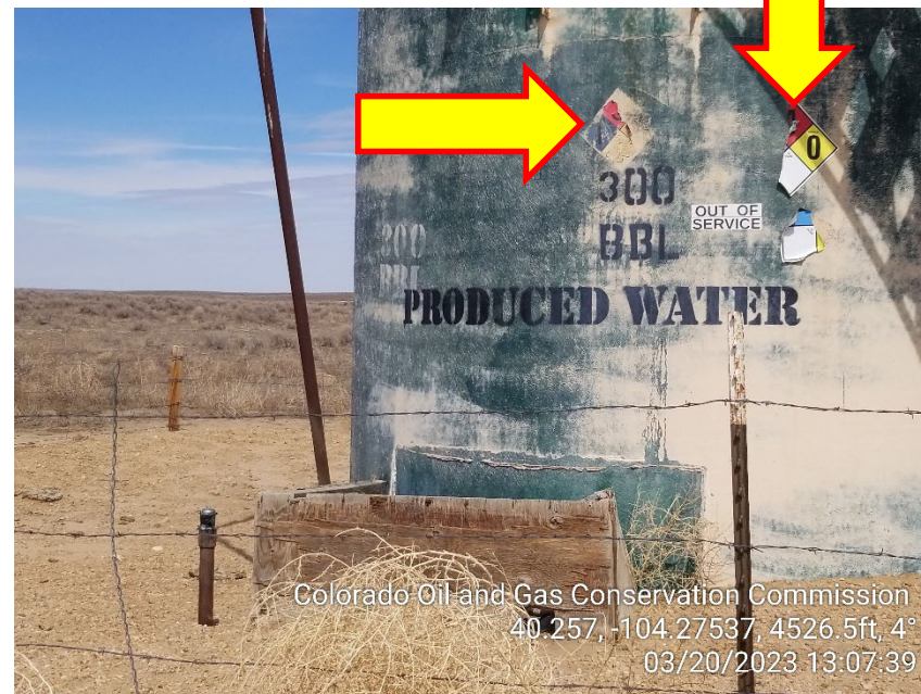
Photo 8 – Produced Water Tank – NFPA Label
