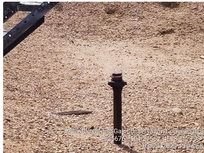
Photo 6 – Unmarked Riser at Crude Oil Tanks
