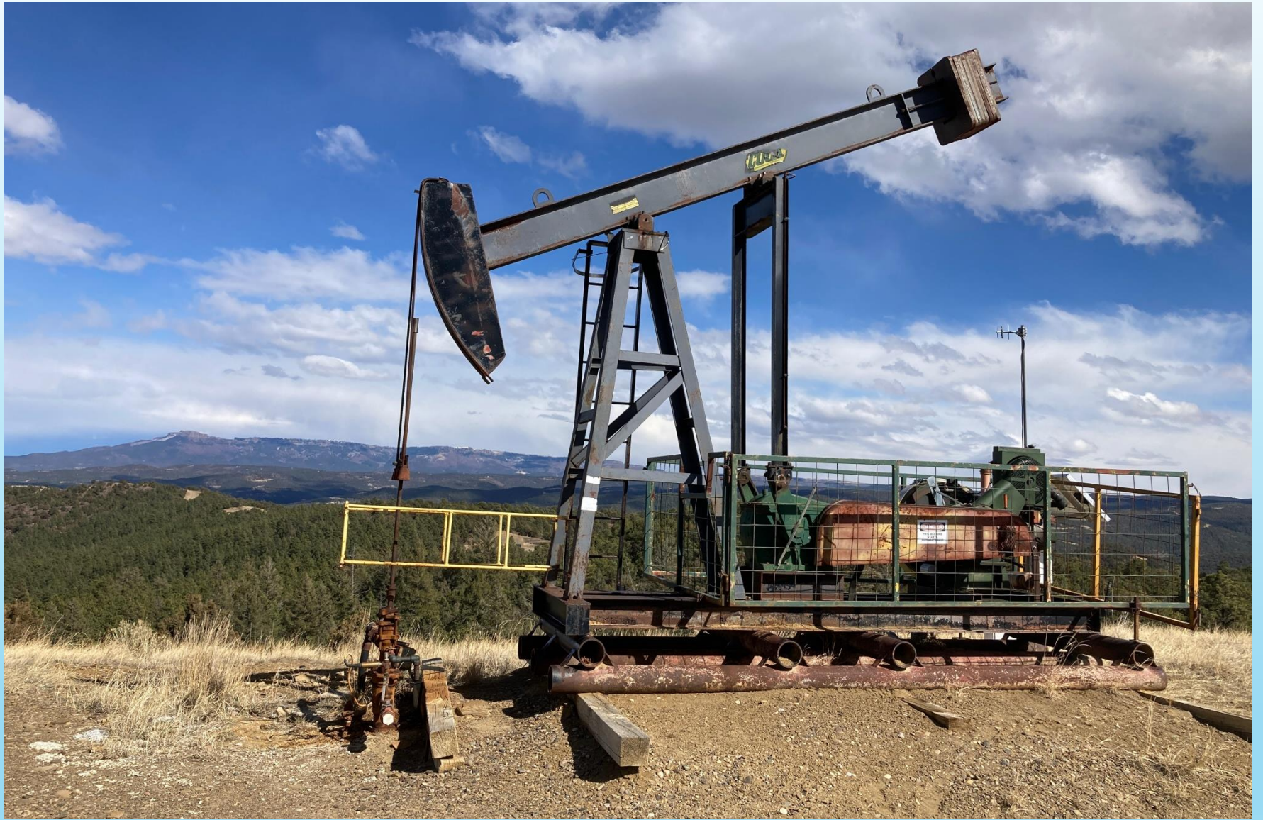
PHOTO 3: WELLHEAD AND EQUIPMENT
