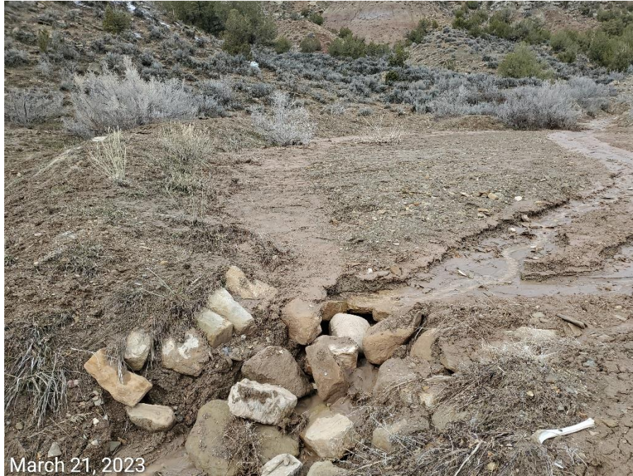
Photo 12: Photos taken from the sediment trap on the west end of the Location. Photo shows BMP appears to have filled with sediment.
