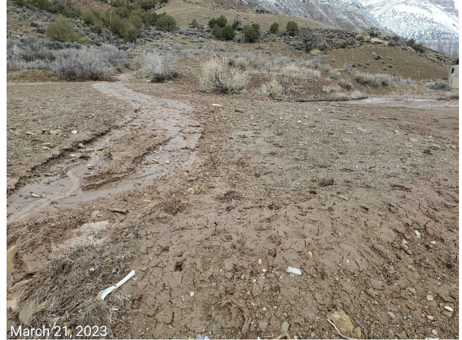
Photo 12: Photos taken from the sediment trap on the west end of the Location. Photo shows BMP appears to have filled with sediment.
