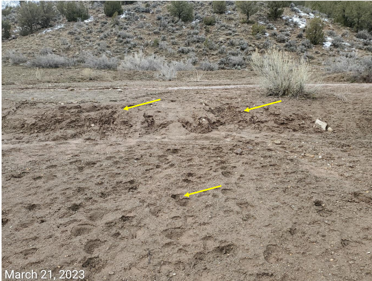
Photo 14: Photo shows areas where stormwater appears to have blown out a section of the sediment trap, resulting in runoff onto the working pad area and sediment deposition.
