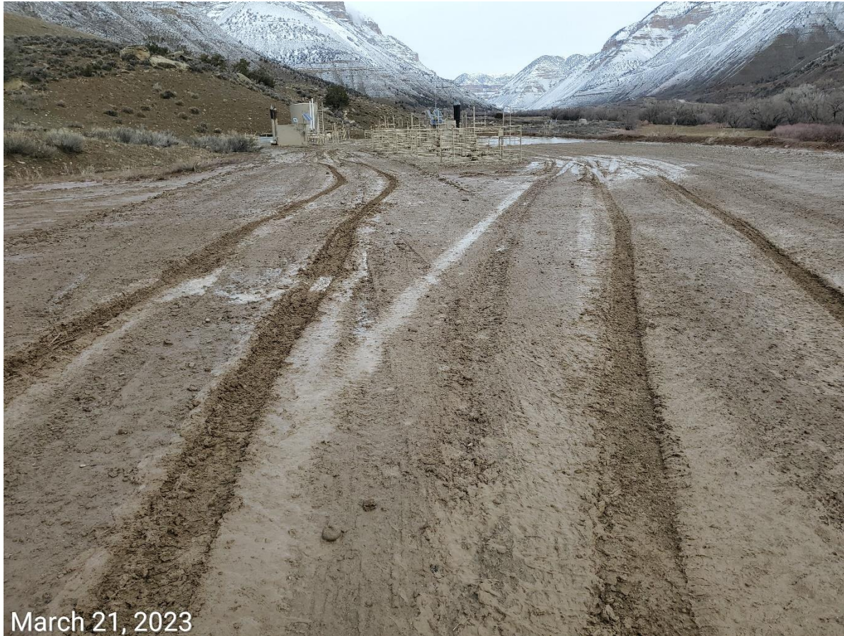
Photo 1: Photos 1-4 taken from the working pad area of the Location. Photos examples showing BMPs, including vehicle tracking control measures, remain missing or insufficient to minimize erosion, degradation, tracking and sediment transport during wet conditions. Regrading alone is inadequate to address tracking and stabilization issues. 6 foot measuring stick for reference.
