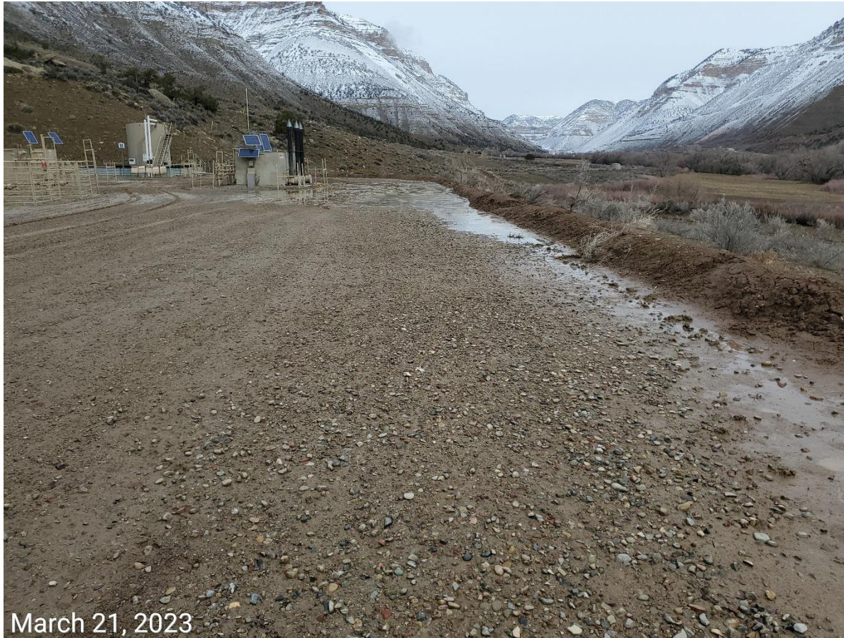
Photo 5: Photo taken from the east end of the Location. Photo shows areas where stormwater is ponding on the east end of the Location. There are several areas where stormwater has blown out the perimeter berm, resulting erosion, degradation, and sediment deposition on top of vegetation of the interim slopes of the Location; Location has not been constructed with an appropriate engineered outlet to allow for proper stormwater discharge.
