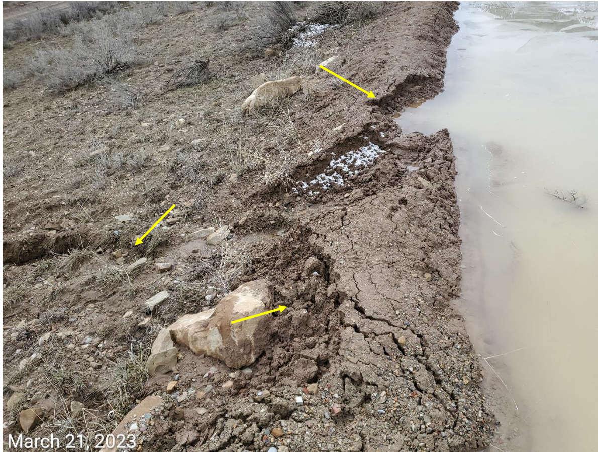
Photo 8: See comments under photo 5. Photo shows areas where stormwater has blown out the perimeter berm, resulting erosion and degradation the interim slopes of the Location; Location has not been constructed with an appropriate engineered outlet to allow for proper stormwater discharge.
