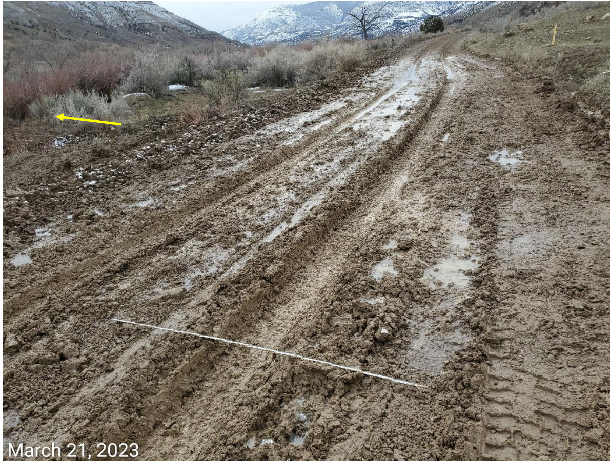
Photo 16: Photo taken example of sections along the main North/South access road, where BMPs to minimize erosion, degradation, tracking and sediment transport remain missing or insufficient. Stormwater does not appear to be being adequately diverted, or discharging from the road. Regrading alone is inadequate to address tracking and stabilization issues. 6 foot measuring stick for reference. Riparian area for Parachute Creek visible in the left of the photo.
