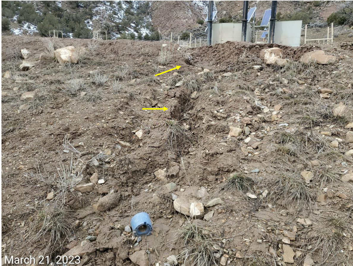
Photo 9: Photo shows stormwater erosion and degradation at the eastern interim slopes of the Location. Location has not been constructed with an appropriate engineered outlet to allow for proper stormwater discharge.
