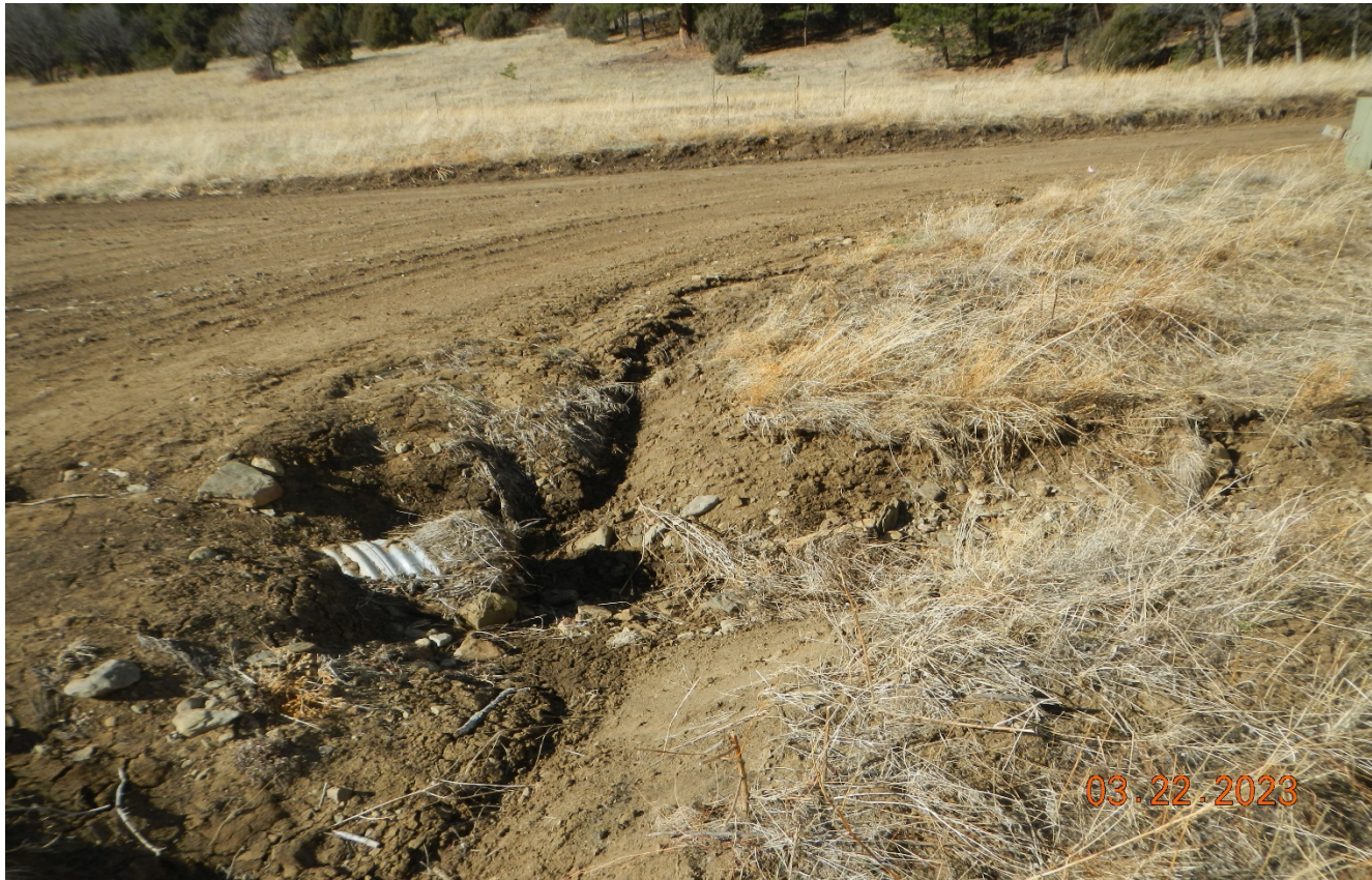
Photo 3. The culvert inlet is filled in with sediment and debris. It appears a larger culvert is needed at this area to handle stormwater coming off the road and drainage. Previous corrective action not completed.
