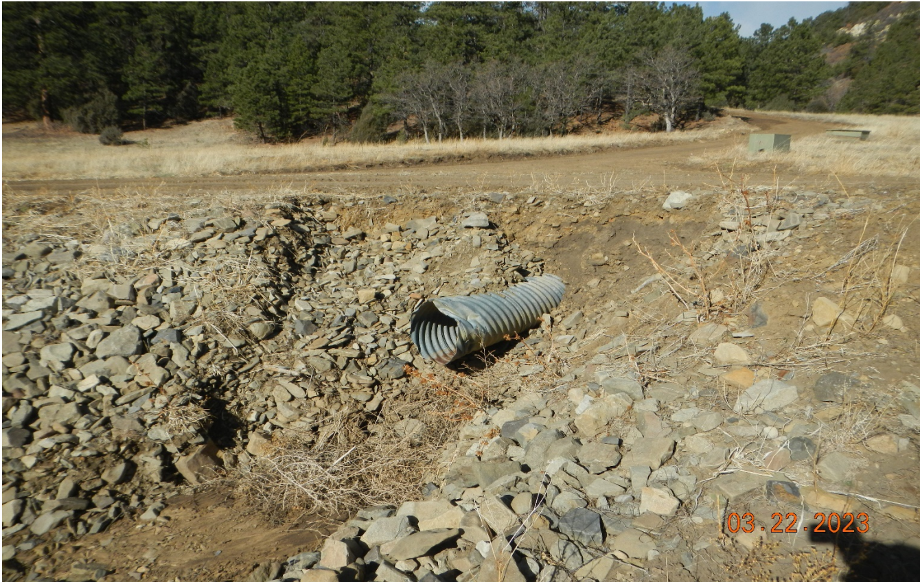
Photo 2. Facing west toward near the access road ascending the hillside. The culvert outlet has been washed out from recent storm event. It appears a larger culvert is needed along with larger rock rip/rap outlet protection. Previous corrective action not completed.
