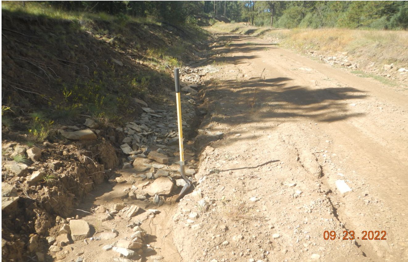
Photo 5. Facing west along the access road. Some of the rock check dams previously installed have washed out. Larger rock was likely needed. A 4.5 ft. shovel shows scale of erosion. Photo taken during previous inspection on 9/23/22.
