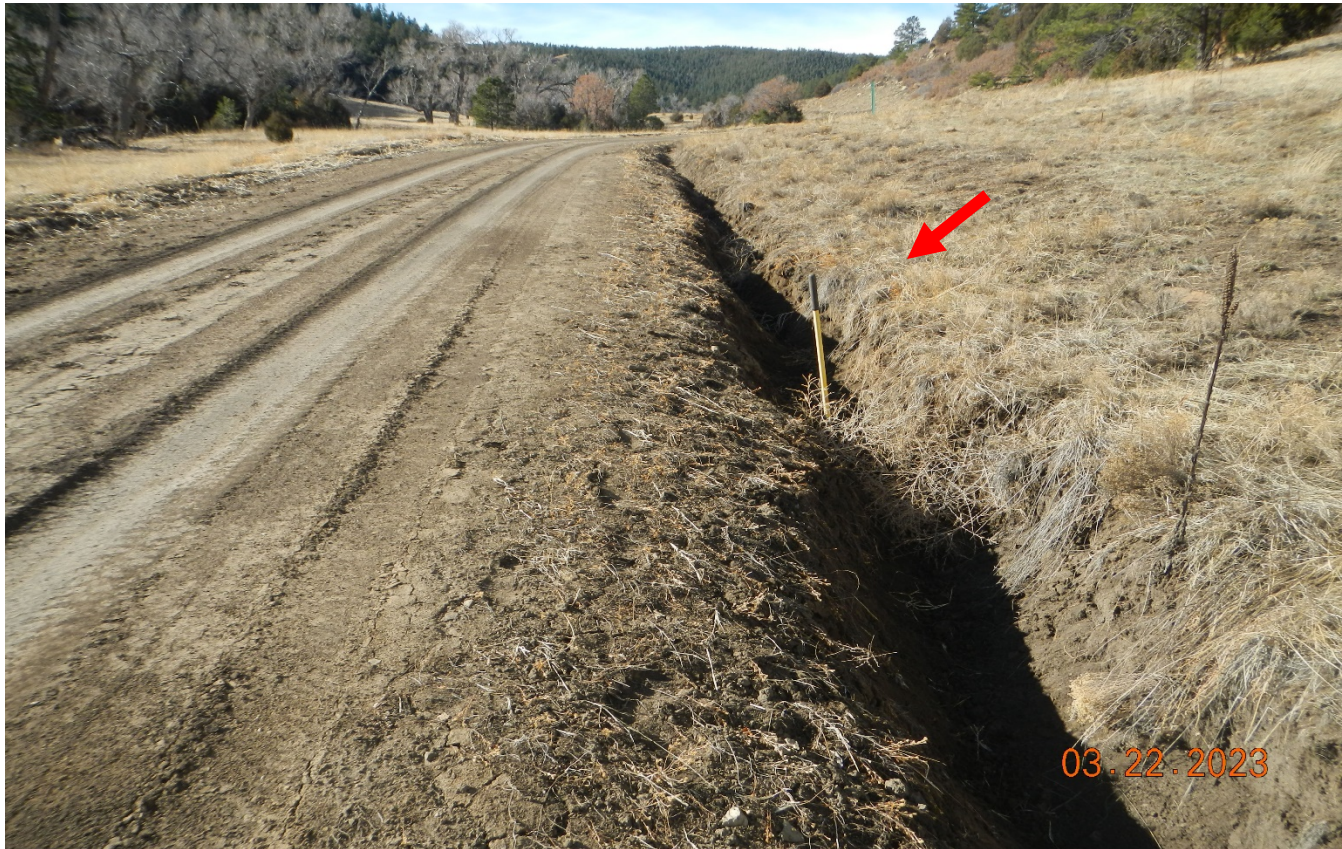
Photo 1. Facing south along the main road. There is erosion occurring along the road side. BMP's need to be installed to prevent erosion. Red arrow points to 4.5' shovel. Previous corrective action not completed.
