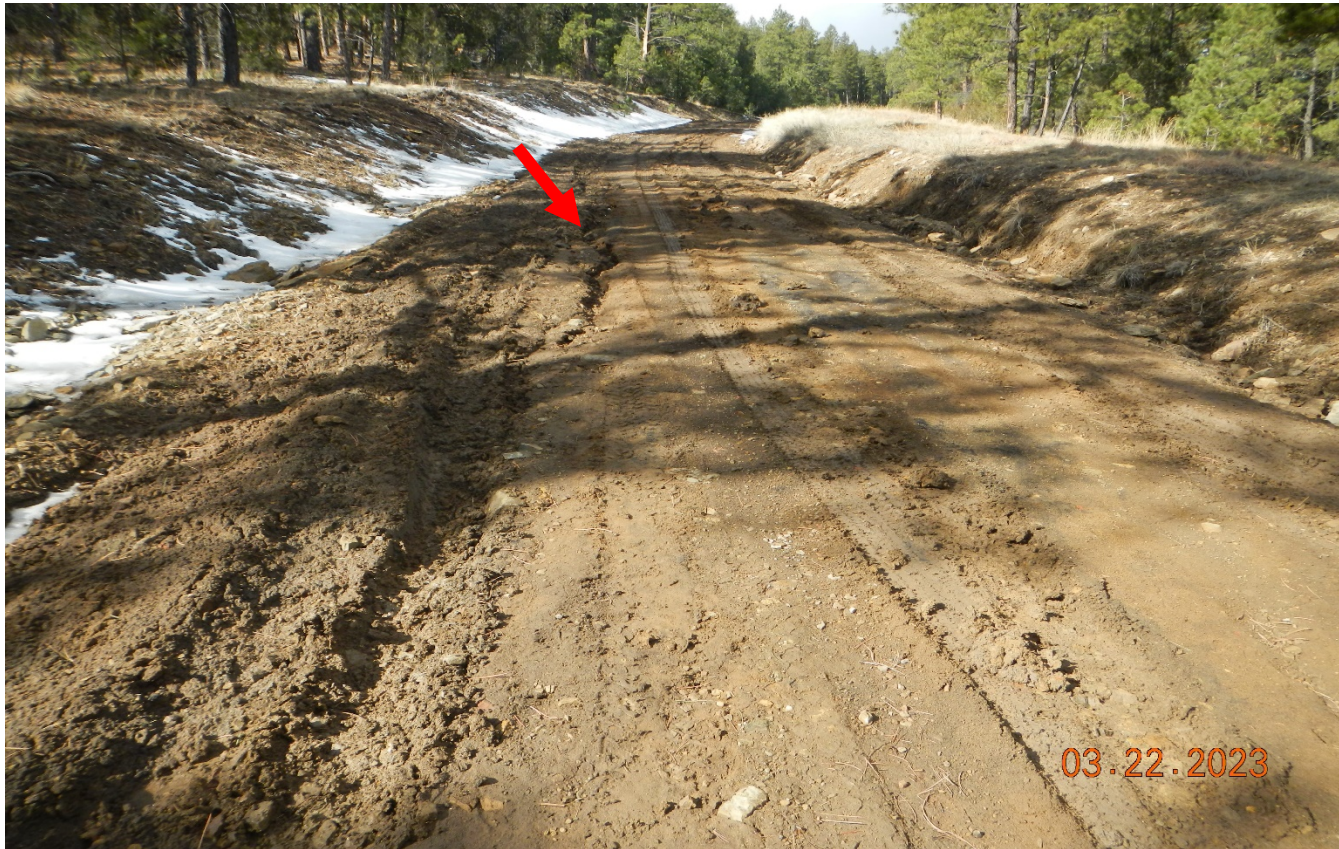
Photo 4. There are signs stormwater is flowing down the road causing erosion. This area has been a problem before and needs to be stabilized. Stormwater is not being properly diverted off the road. Additionally the road is very slick and vehicle rutting is occurring.
