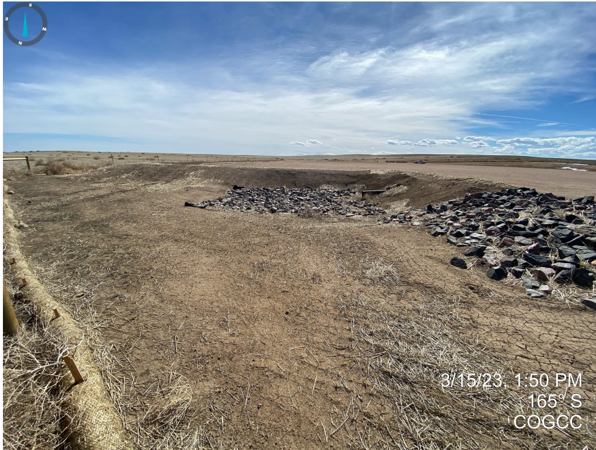
Photo 6. Facing south from the eastern/center portion of the location. Operator installed a sediment trap with a rip-rap structure to stabilize the outlets and protect against erosion. Straw wattles were also observed around the entire perimeter of the location and appear to be properly installed per good engineering practices.
