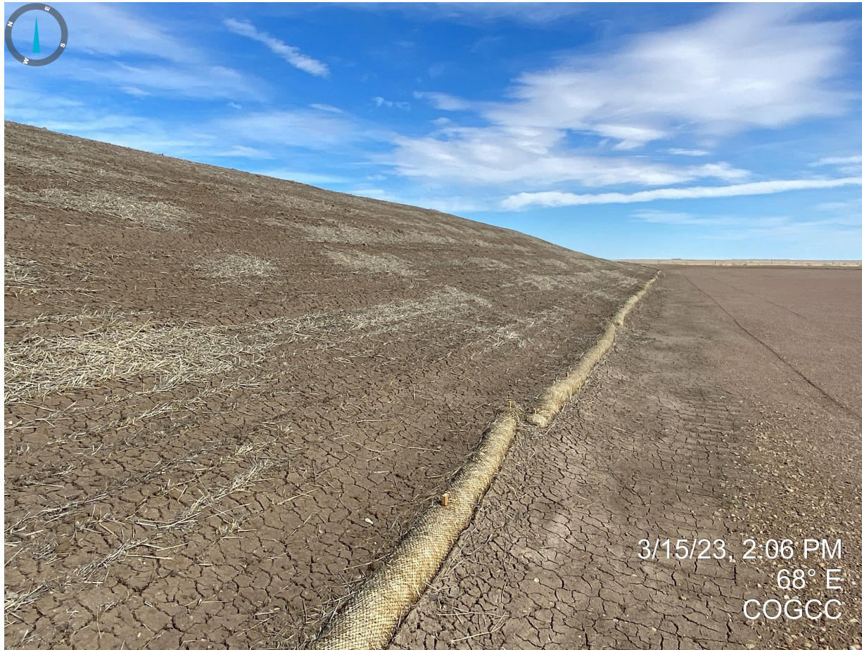
Photo 7. Facing east near the topsoil stockpile. It appears the operator has salvaged all of the topsoil from the disturbance area and stored it on the northern end of the location. Straw wattles were observed around the entire perimeter of the stockpile.
