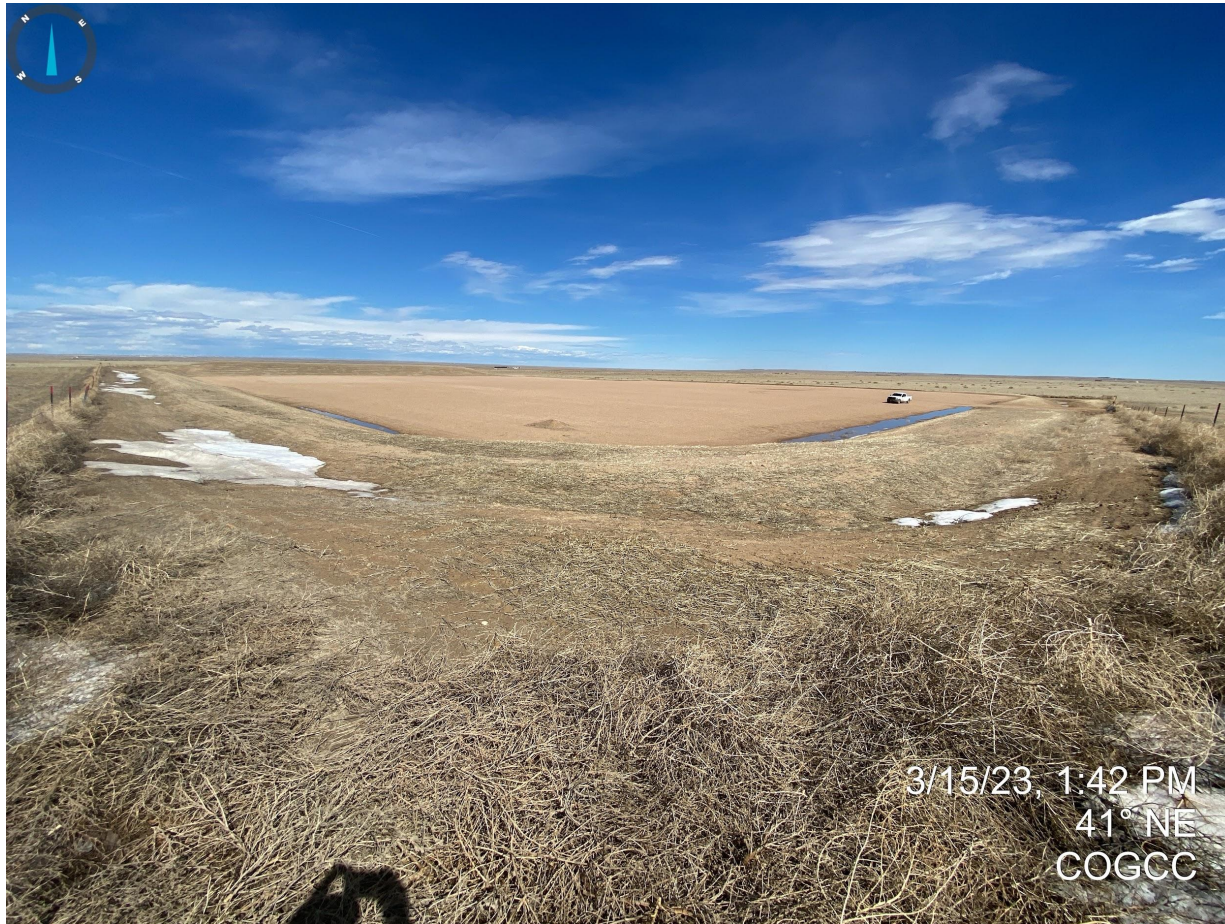
Photo 2. Facing northeast from the southwest corner of the location. Perimeter ditch and berm has been installed during the construction phase of the location. These areas appeared to have been stabilized as crimped straw mulch and drill rows were evident.
