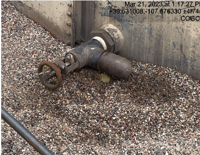
Staining under valve
