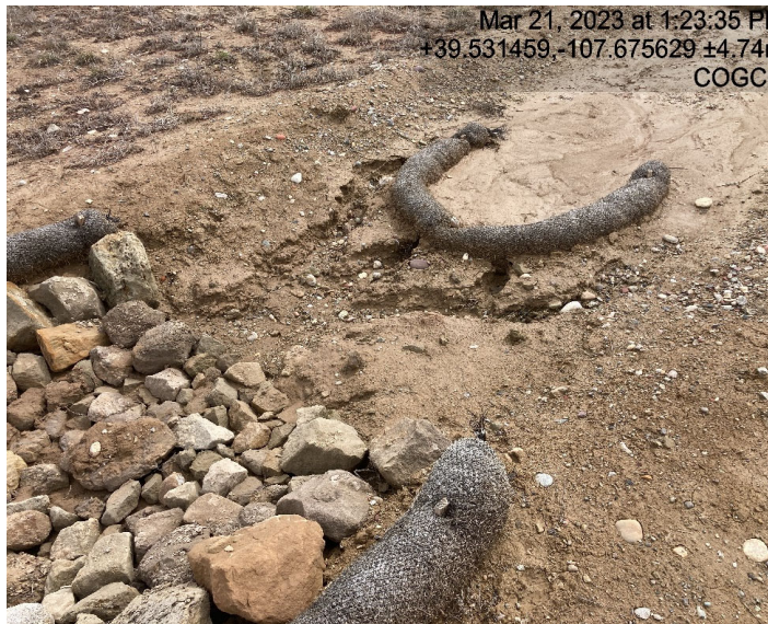
Erosion under waddles
