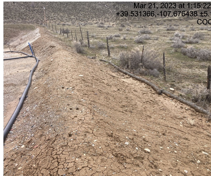
Fill slope shows lack of stabilization
