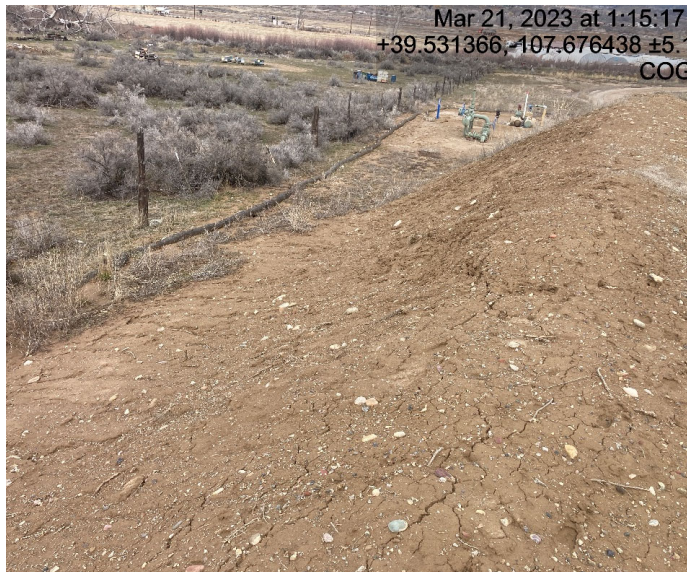
Fill slope shows lack of stabilization
