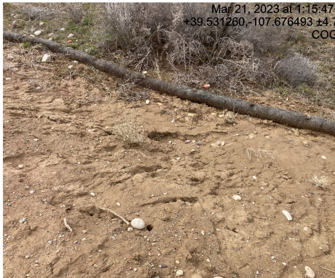
Erosion is undermining location berm coming out of fill slope
