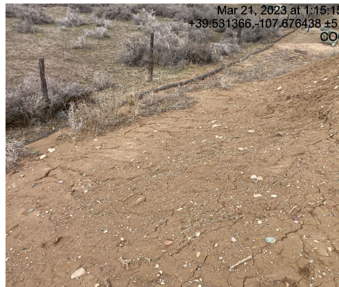
Fill slope shows lack of stabilization
