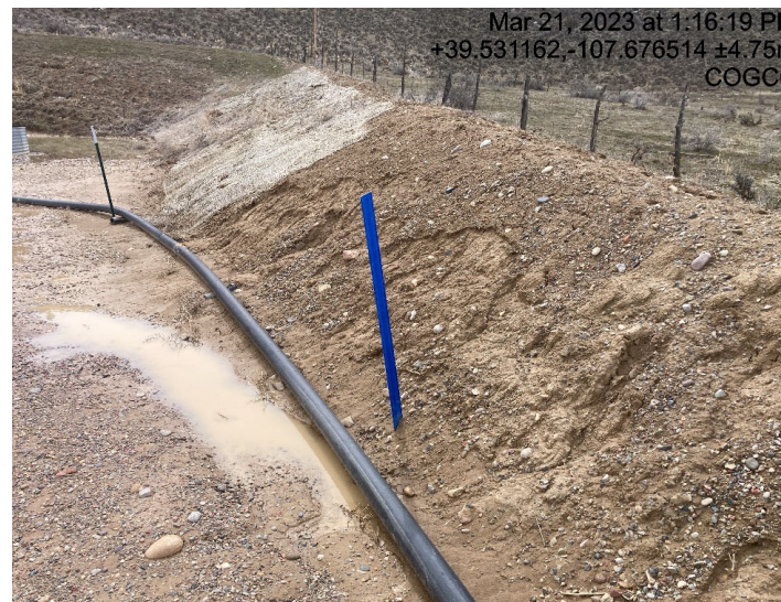
Cut slope shows signs of erosion, Blankets have been installed in areas.
