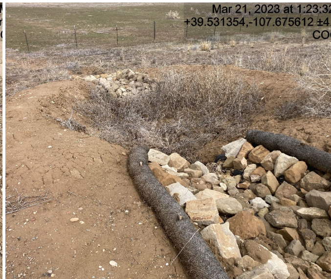
Sediment trap full of weeds
