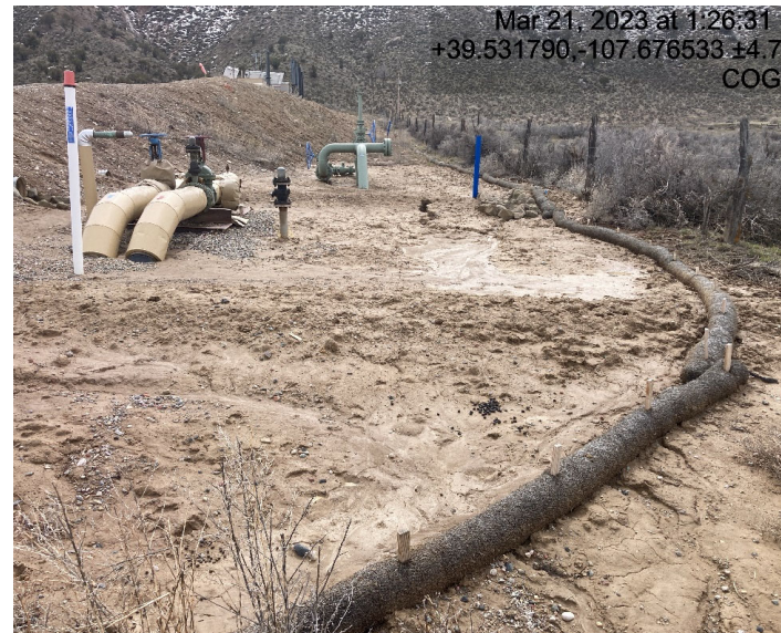
Multiple areas of erosion next to access road with BMP's failing
