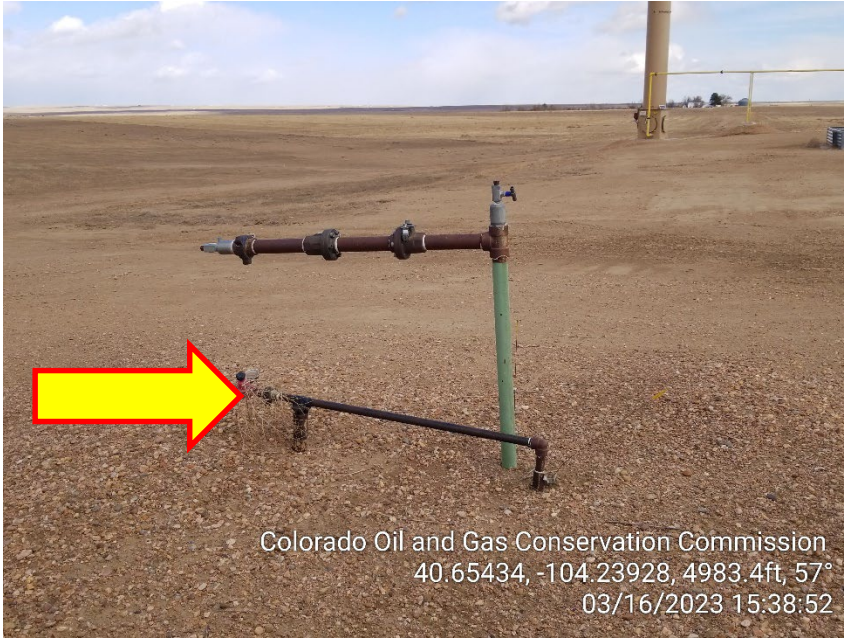
Photo 5 – Unmarked Riser
