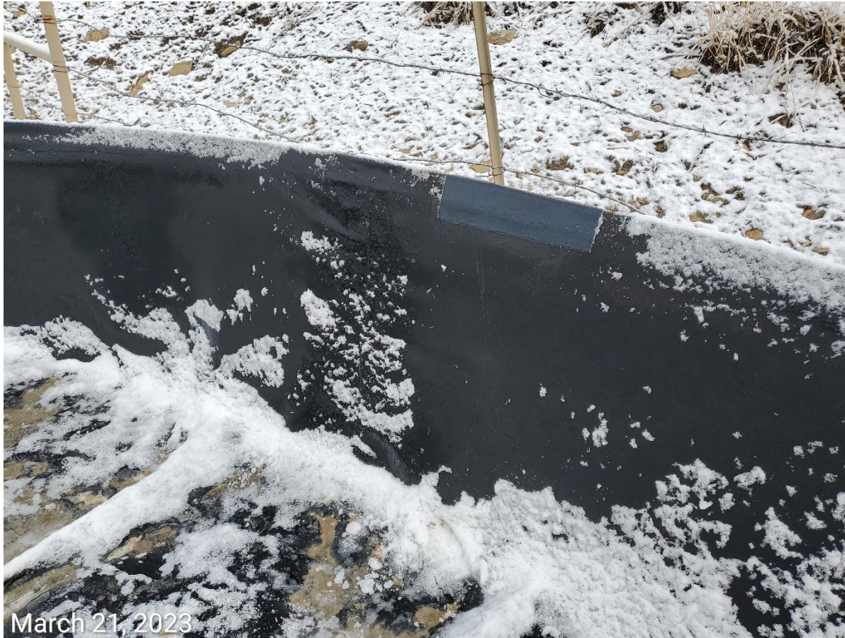
Photo 4: Photo taken from the tank battery. Photo shows repairs appear to have been made to the secondary containment liner.
