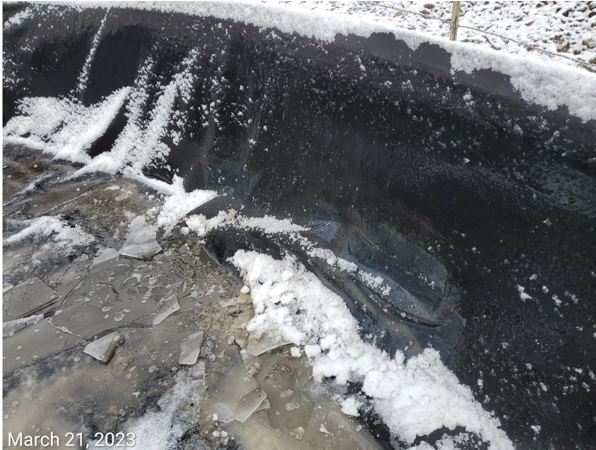
Photo 6: Photo shows liner appears to have been repaired.
