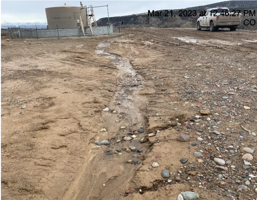
Photo # 2763 – Rill erosion/ditch needs maintenance
