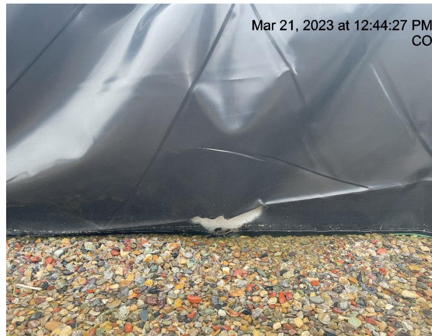
Photo # 2759 Containment liner needs maintenance
