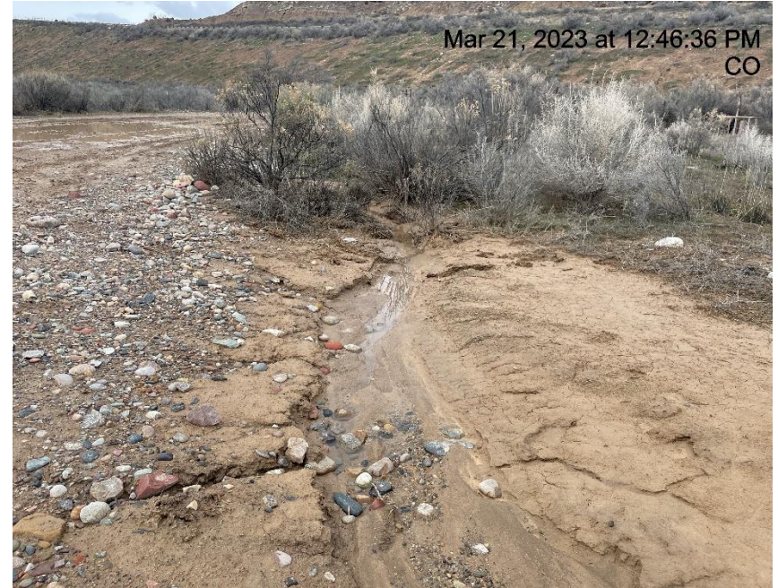
Photo # 2764 Rill erosion/ditch needs maintenance
