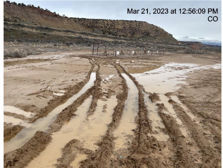
Photo # 2795 Lack of stabilization
