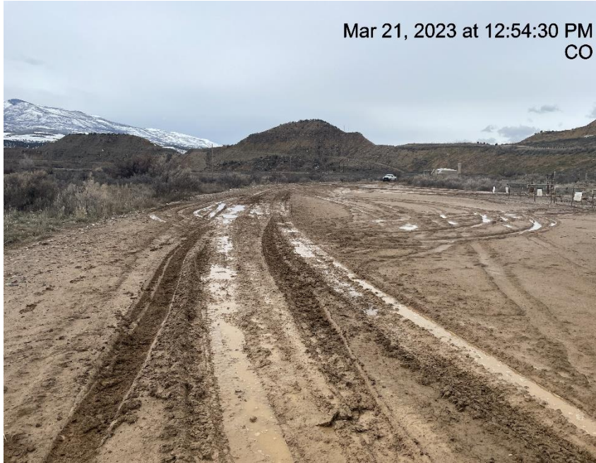
Photo # 2789 Lack of stabilization
