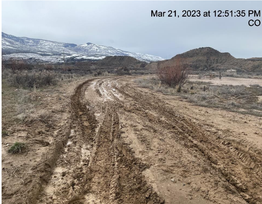
Photo # 2775 Lack of stabilization
