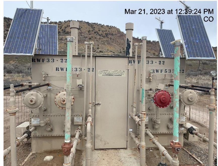
Photo # 2750 Meter calibration info not conspicuously posted
