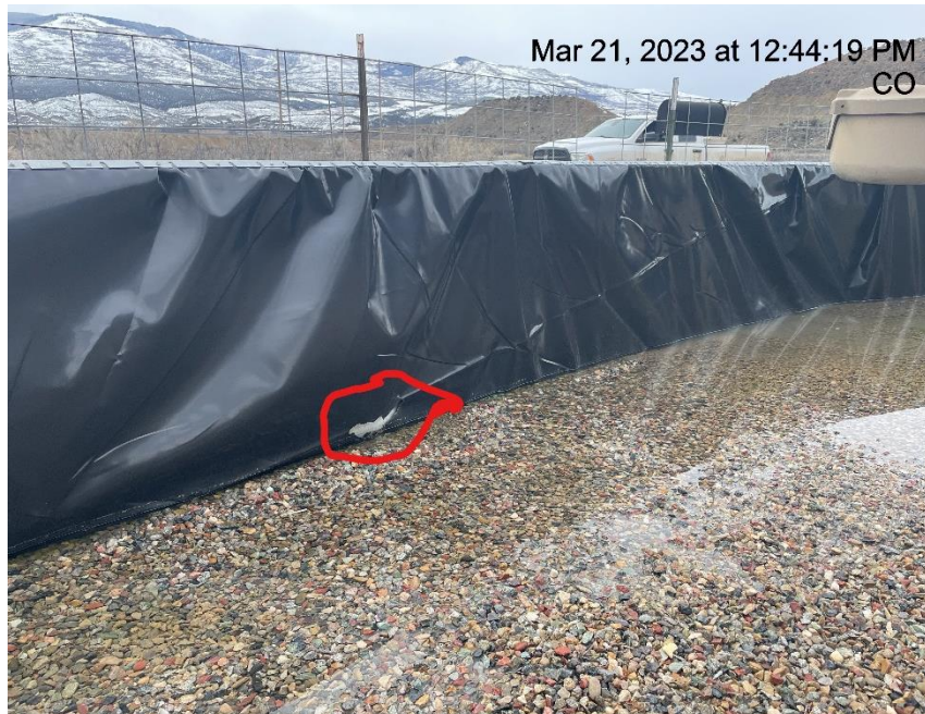
Photo # 2758 Containment liner needs maintenance
