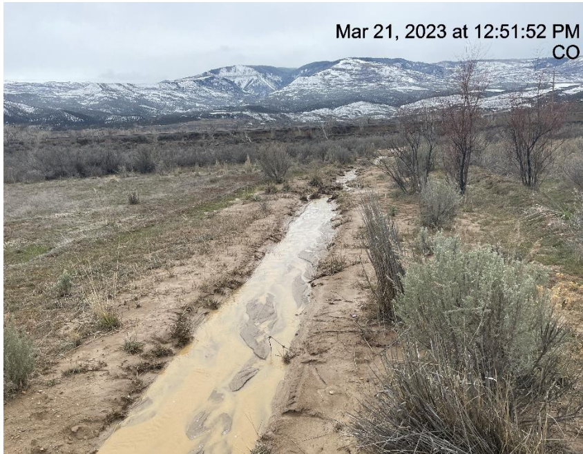
Photo # 2776 Ditch needs maintenance (E/SE side of location)
