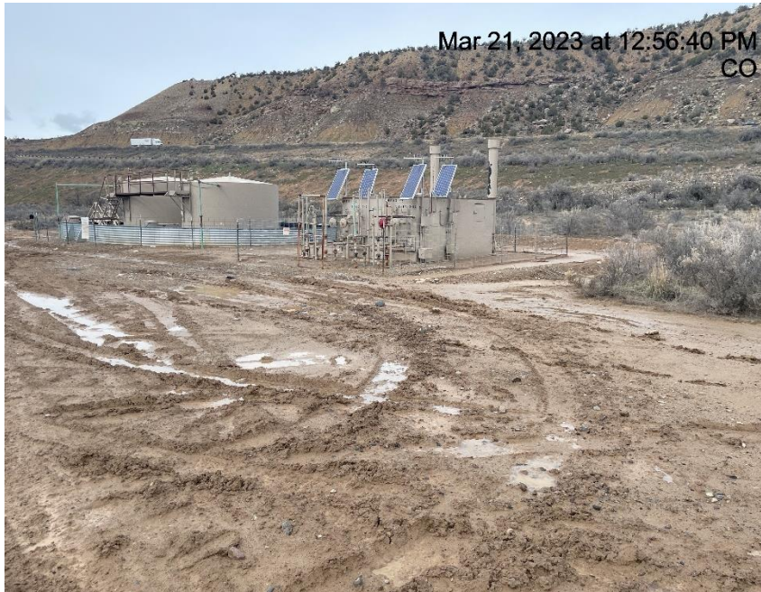
Photo # 2797 Lack of stabilization
