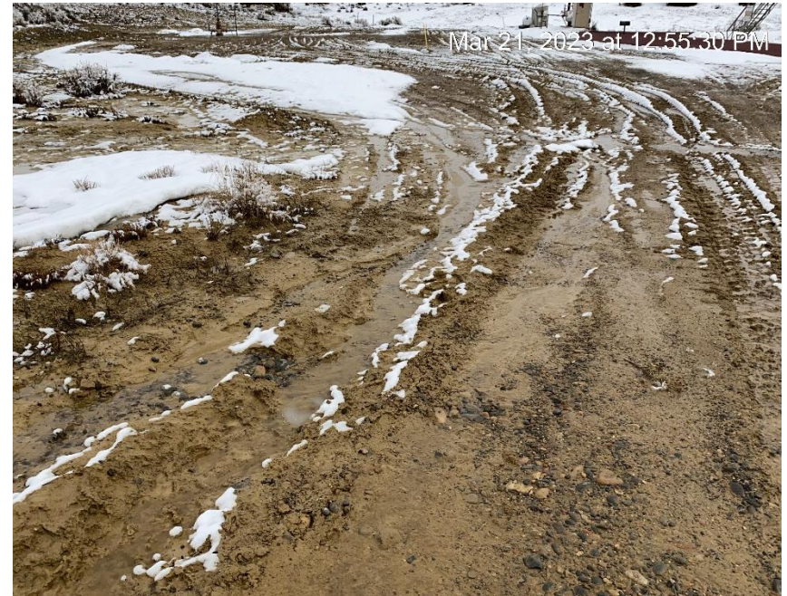
Drainage ditch allowing sediment migration off location
