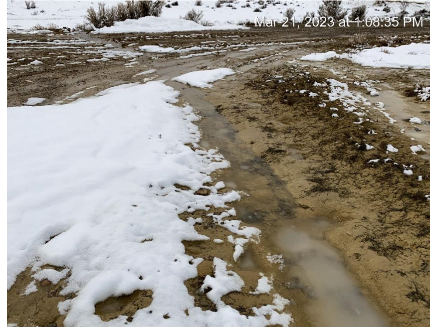
No BMP to prevent sediment migration off location
