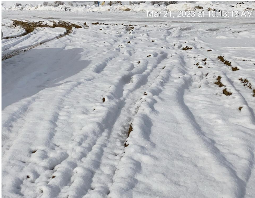
No South entrance vehicle tracking BMP installed
