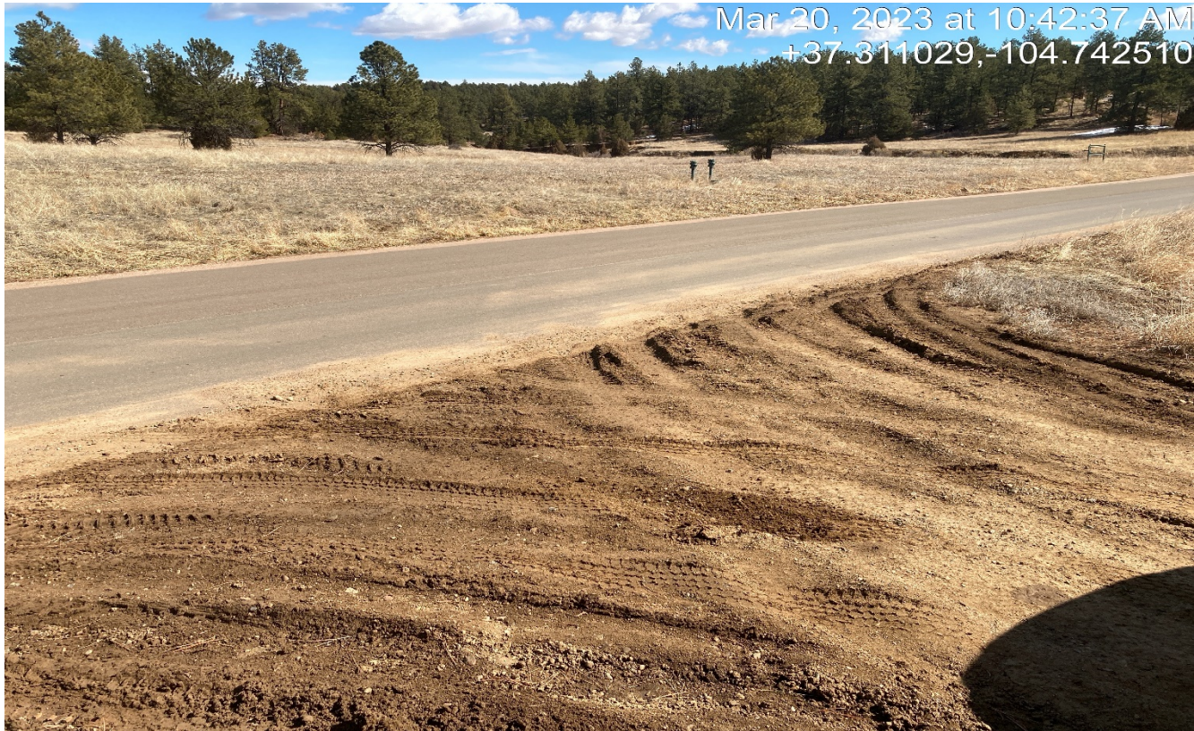
Photo 2. There is signs of vehicle tracking onto the county road.
