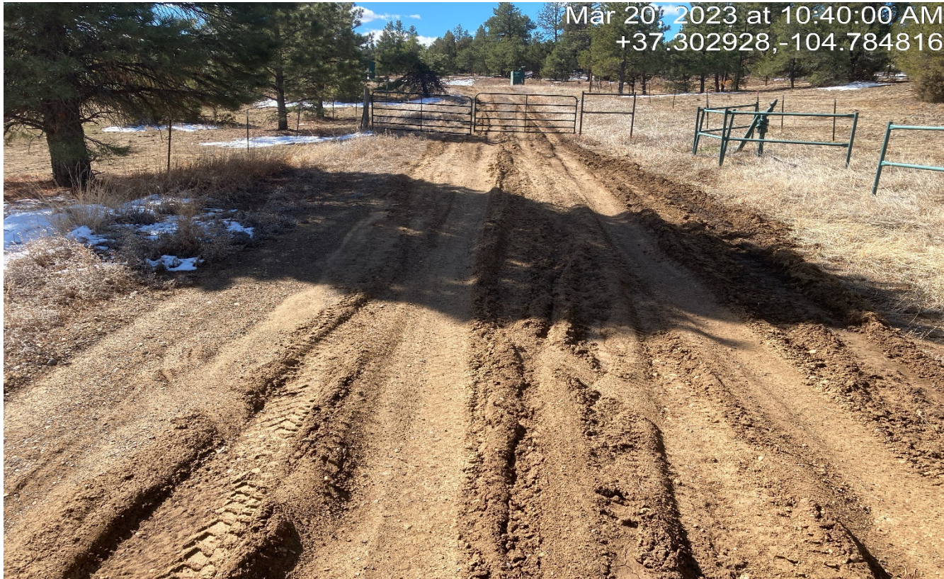
Photo 1. Facing south toward the access road. There are vehicle ruts and the road is not compacted and stabilized.
