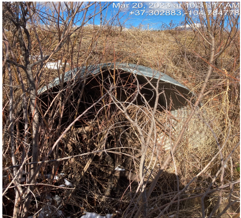
Photo 1. The culverts at the creek crossing along the main road are filled in with debris restricting water flow. Culverts need to be cleaned out.
