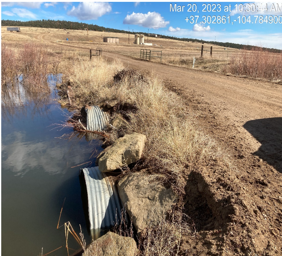
Photo 1. The culverts at the creek crossing along the main road are filled in with debris restricting water flow. Culverts need to be cleaned out.
