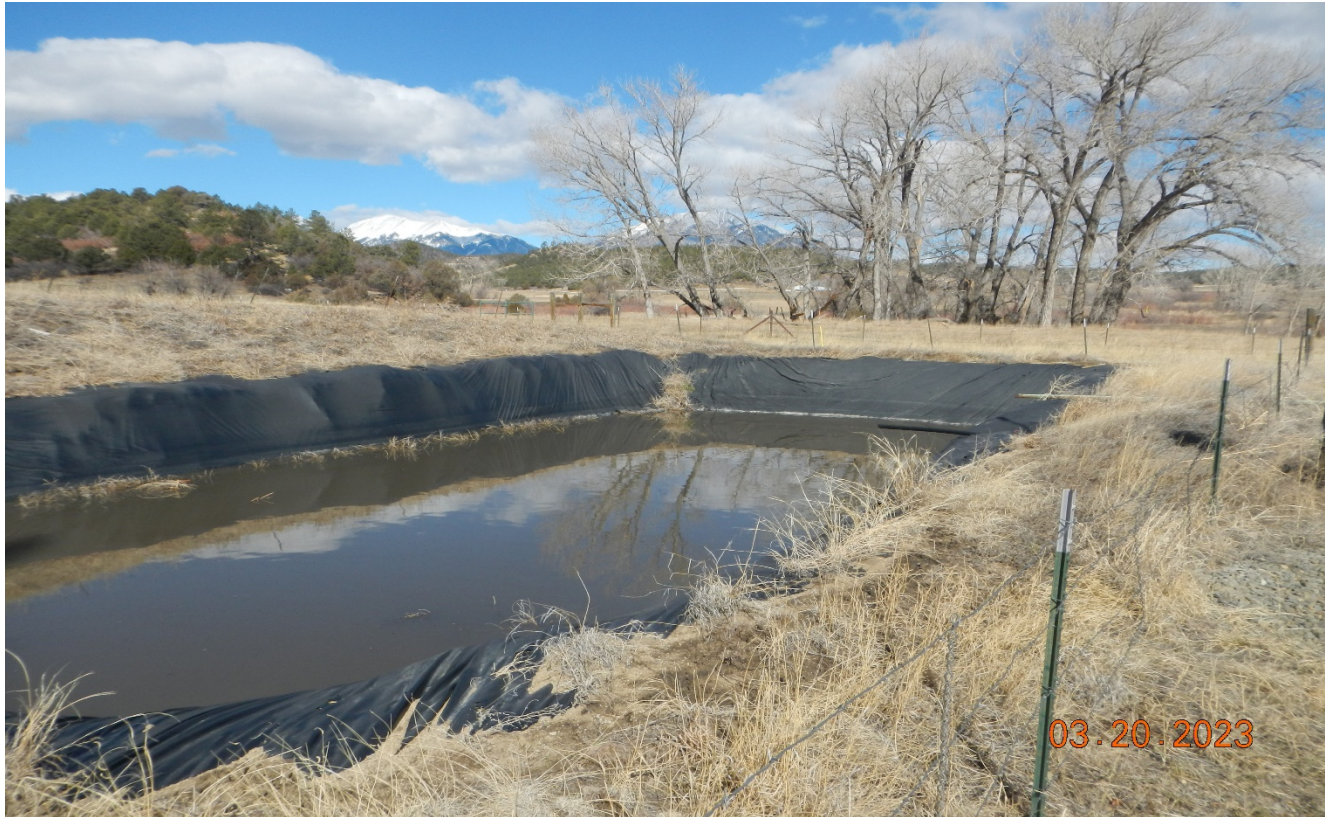
Photo 4. The pit liner still remains torn and water has not been lowered.
