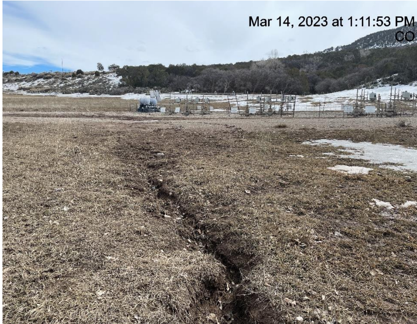
Photo # 2405 Gulley erosion off edge of pad
