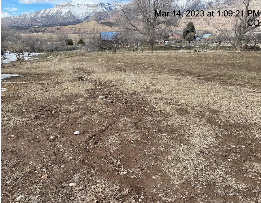
Photo # 2400 Gulley erosion off edge of pad
