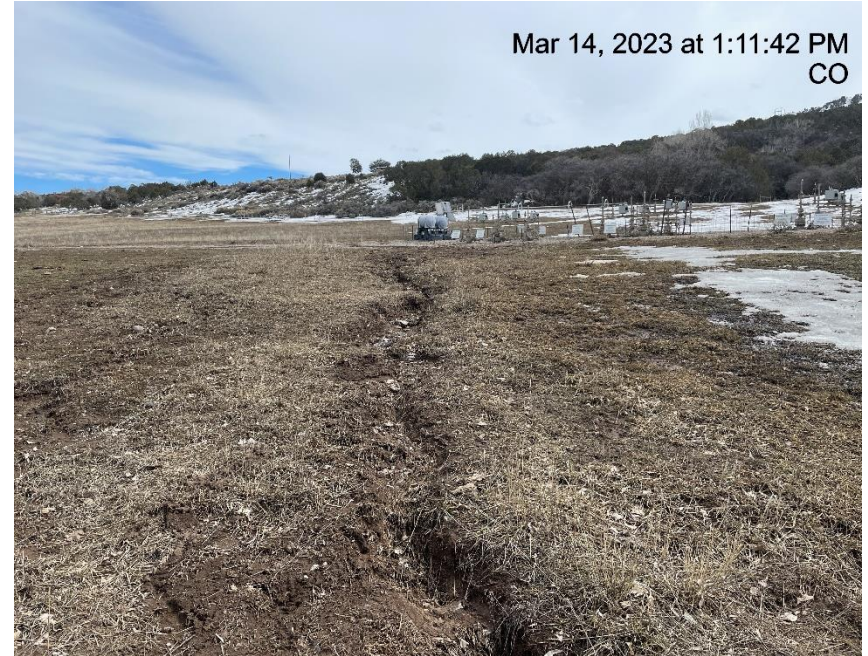
Photo # 2404 Gulley erosion off edge of pad
