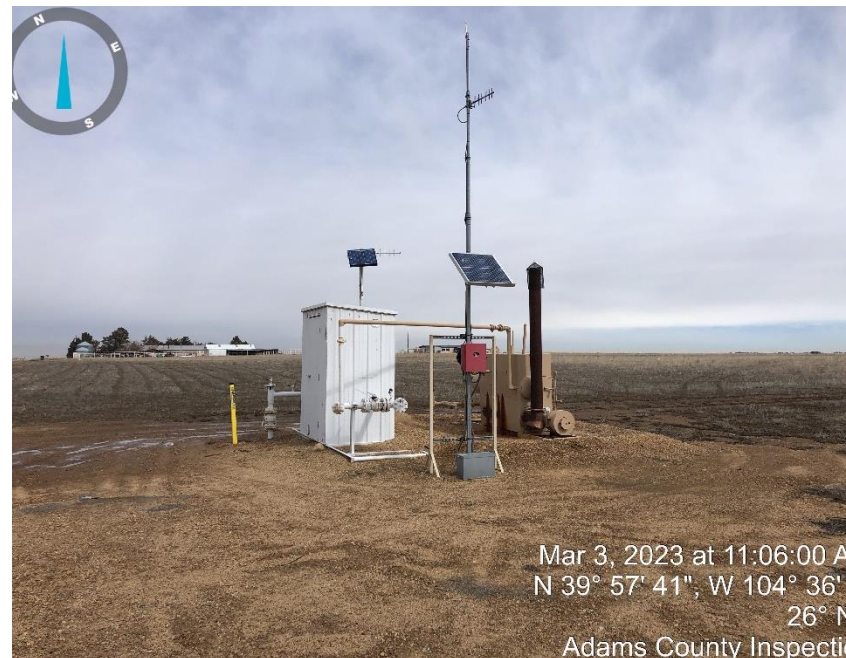
Photo# 2 Separator & Meter.
