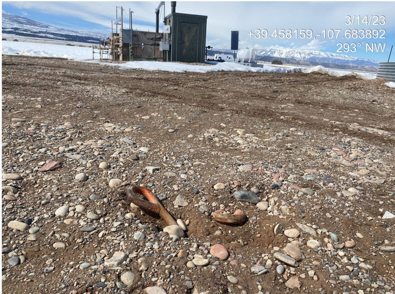
Photo 3. Photos shows two (2) unmarked anchors.
