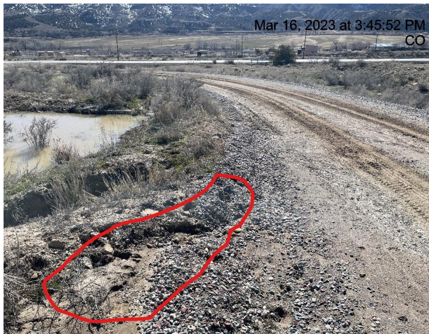
Photo # 2564 Ditch needs maintenance (Access road)
