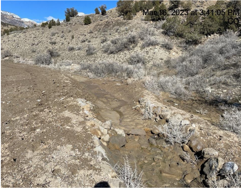
Photo # 2554 Rip Rap needs maintenance (SW corner of location)
