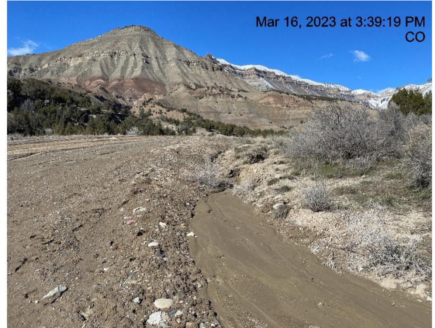
Photo # 2550 Ditch needs maintenance (SE corner of location)
