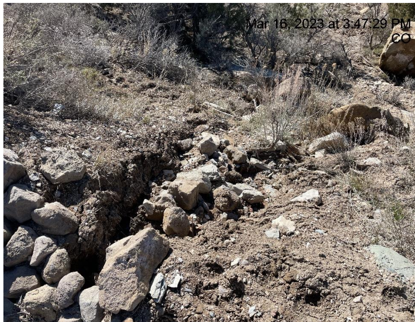
Photo # 2567 Sediment Trap needs maintenance (N side of location off access road)
