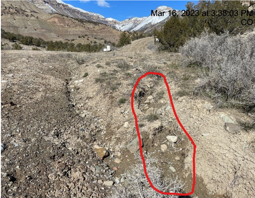
Photo # 2549 Gulley erosion into ditch (SE corner of location near road)
