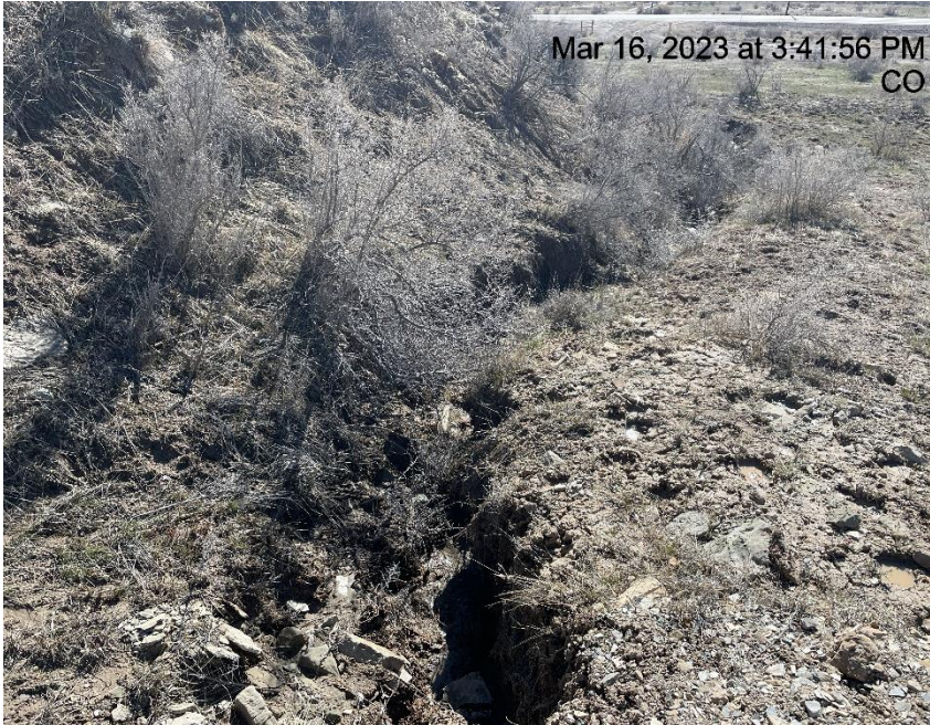
Photo # 2556 Insufficient runoff controls/BMP's – Channel erosion (SW corner of location)
