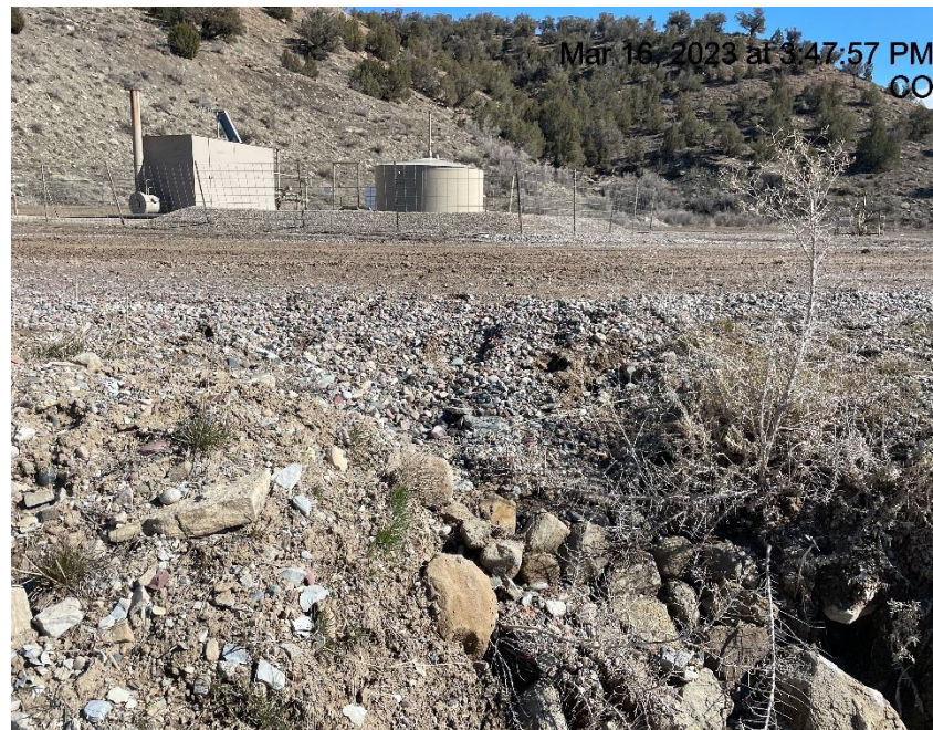
Photo # 2569 Sediment Trap needs maintenance (N side of location off access road)
