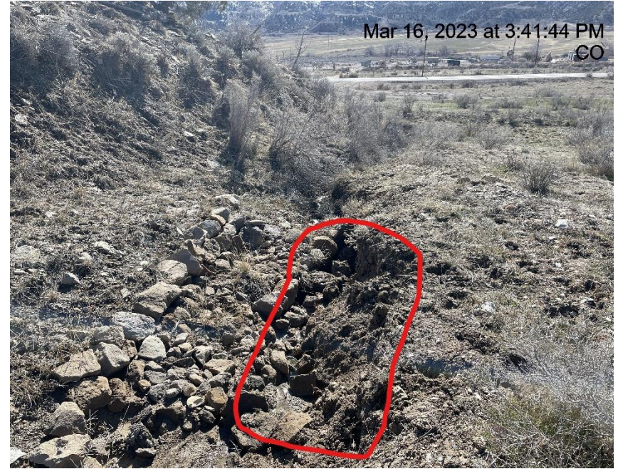
Photo # 2555 Rip Rap needs maintenance (SW corner of location)
