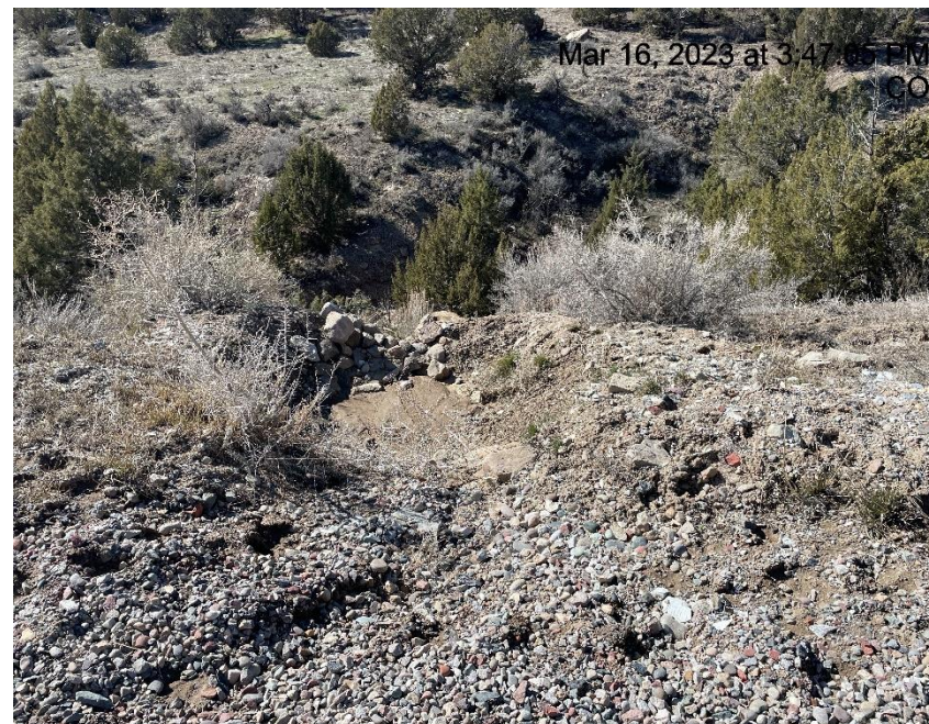
Photo # 2565 Sediment Trap needs maintenance (N side of location off access road)
