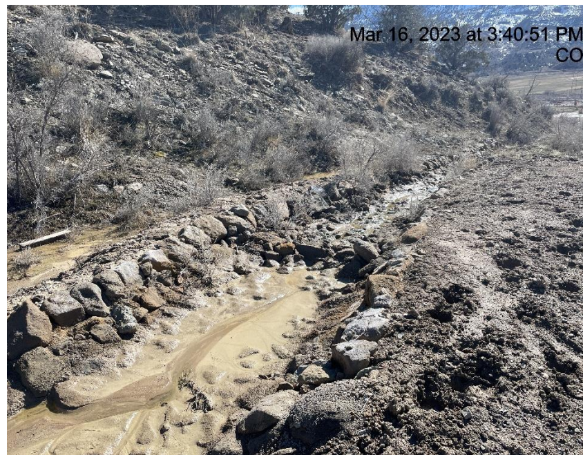
Photo # 2553 Rip Rap needs maintenance (SW corner of location)
