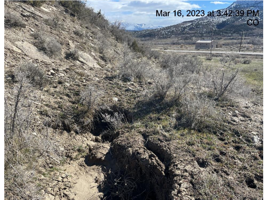
Photo # 2560 Insufficient runoff controls/BMP's – Channel erosion & berm needs maintenance (off SW corner of location)
