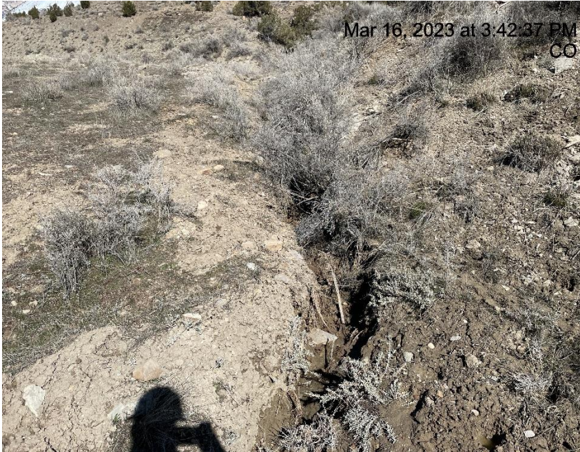
Photo # 2559 Insufficient runoff controls/BMP's – Channel erosion (off SW corner of location)
