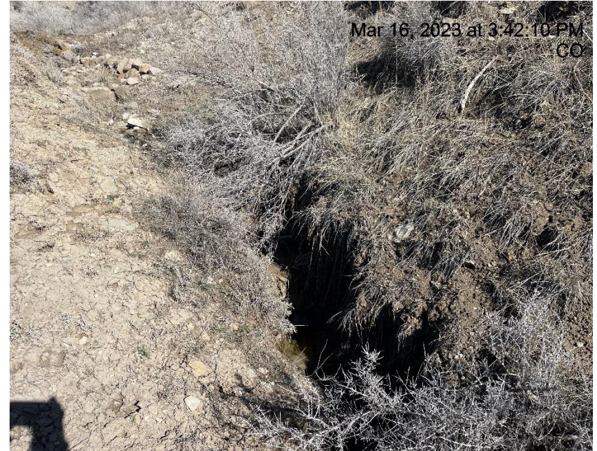
Photo # 2557 Insufficient runoff controls/BMP's – Channel erosion (off SW corner of location)
