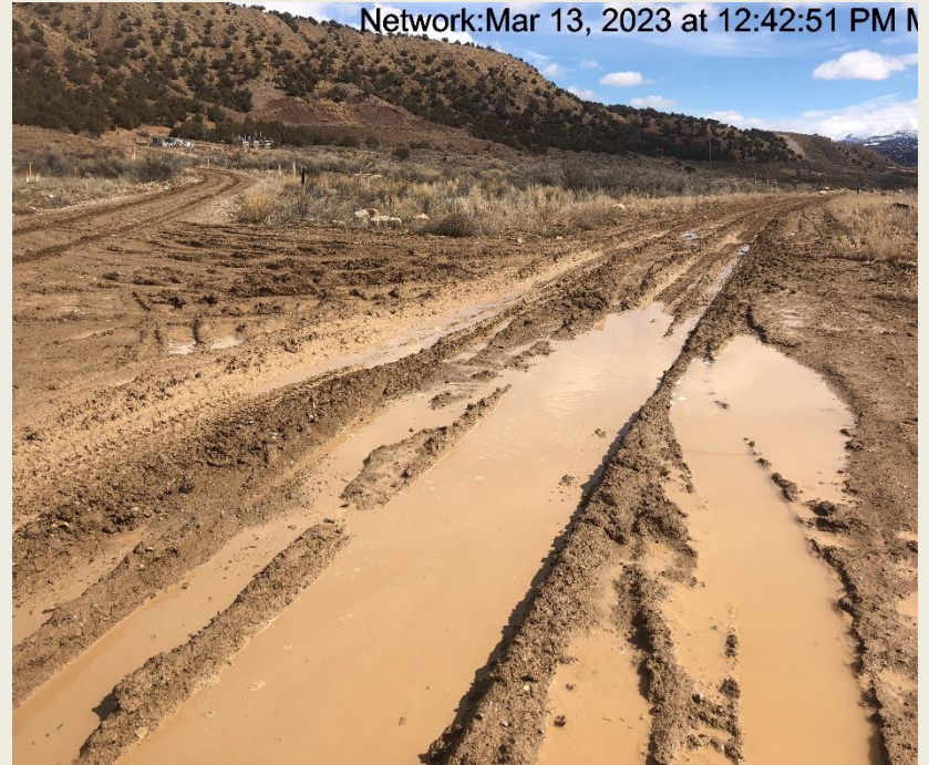
Photo #9230 Insufficient tracking BMP at entrance to access road.
