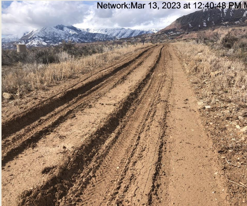
Photo #9229 Access road lacks stabilization.
