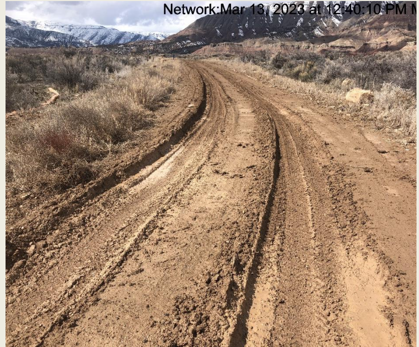
Photo #9228 Access road lack stabilization.
