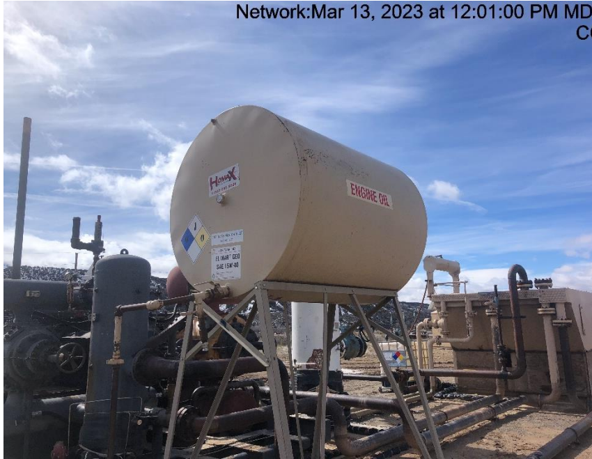
Photo #9211 Multiple tanks missing required information.
