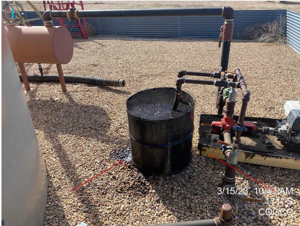
Photo 1. Facing south within secondary containment of battery. Oily waste/stained soil observed around barrel was identified in previous inspection (Doc #696105742) and has not been addressed. The corrective action is being back-dated to when it should have been addressed (see attached report for details).
