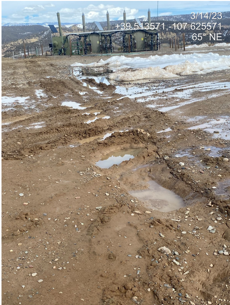
Photo 3. Photos show recently disturbed soils. The working pad is not stabilized.
