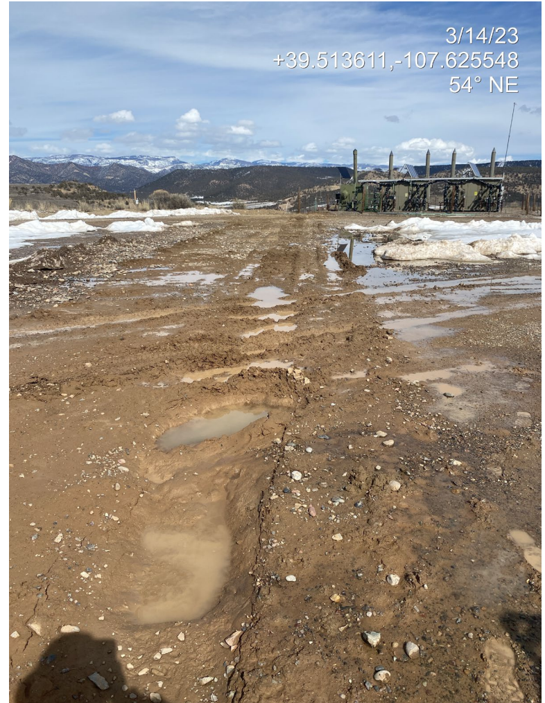
Photo 3. Photos show recently disturbed soils. The working pad is not stabilized.
