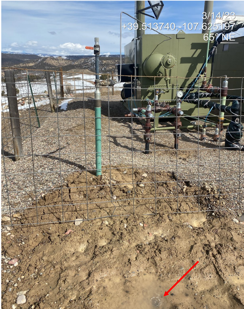
Photo 2. Photos show bubbles rising in the area of a separator and flowline.
