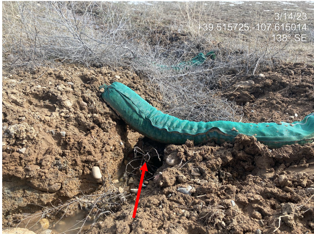
Photo 2. Photos show stormwater cutting beneath velocity check dams and eroding a stormwater ditch.
