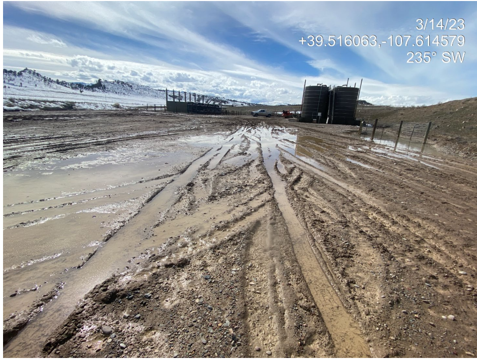
Photo 1. Photos show degradation to the pad surface and lack of stabilization BMPs and tracking controls.
