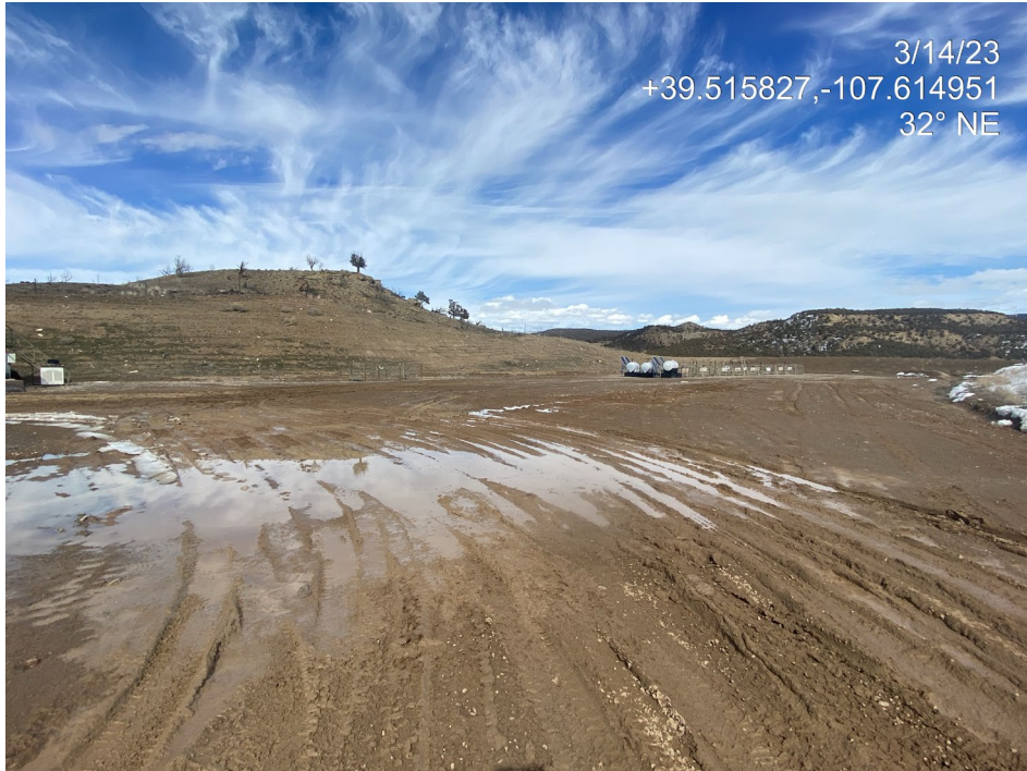
Photo 1. Photos show degradation to the pad surface and lack of stabilization BMPs and tracking controls.
