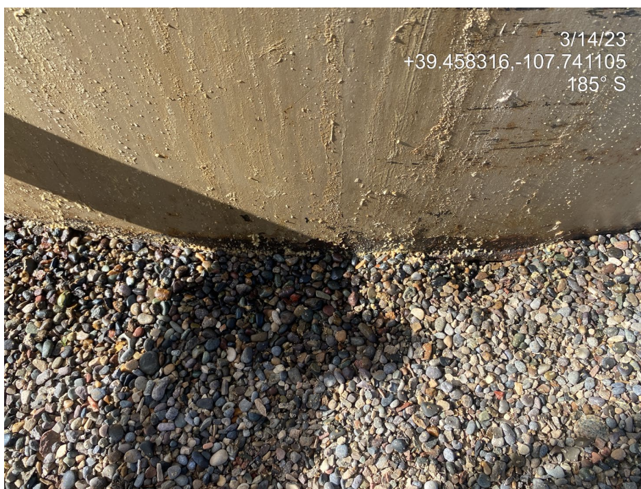
Photo 2. Photos show stained gravel in secondary containment below spilled produced water/condensate tank # 81396.
