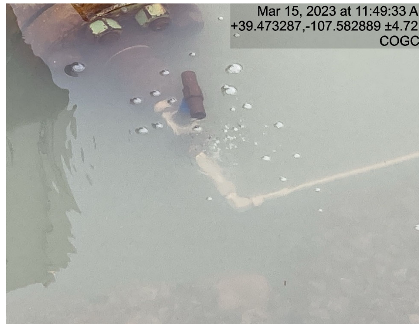
Chemical line leaking
