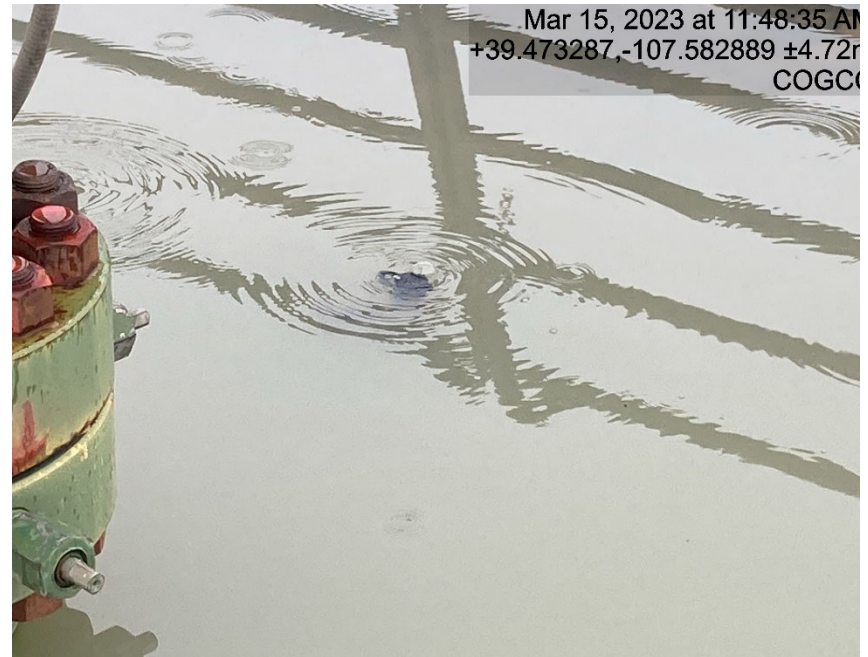
Braden head line leaking
