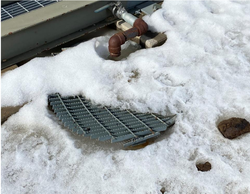
Catch tank cover not properly installed
