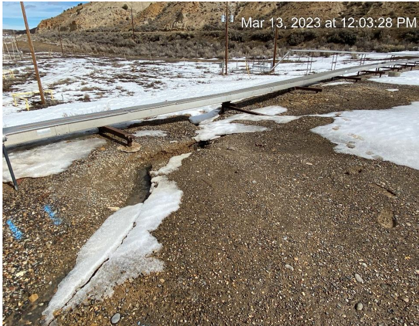
Water exiting location causing erosion
