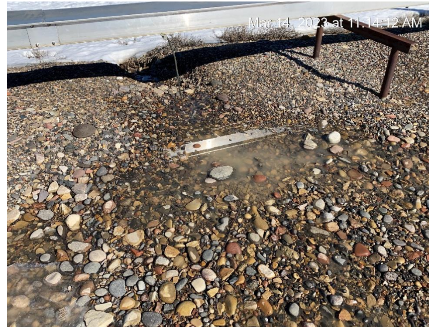
Water leaving location causing erosion
