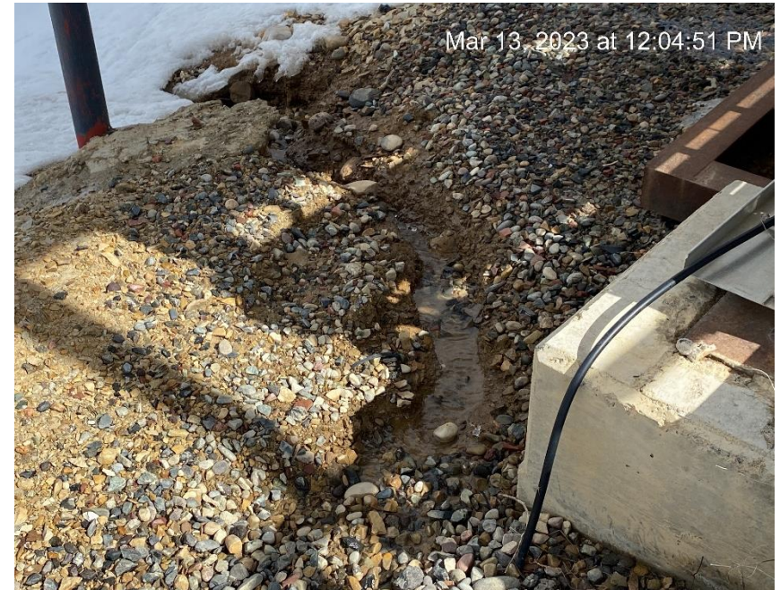
Water exiting location causing erosion
