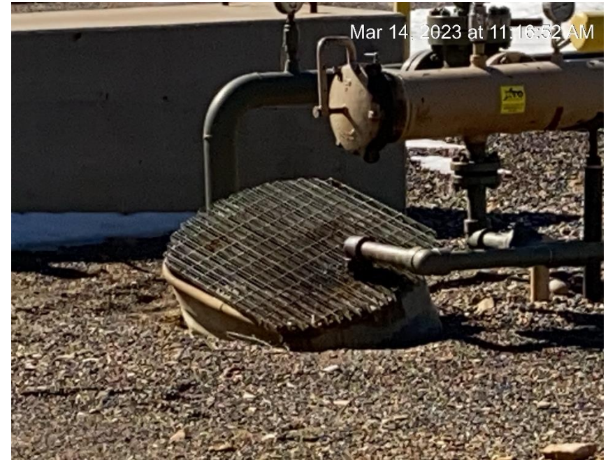
Lack of maintenance, catch can full
