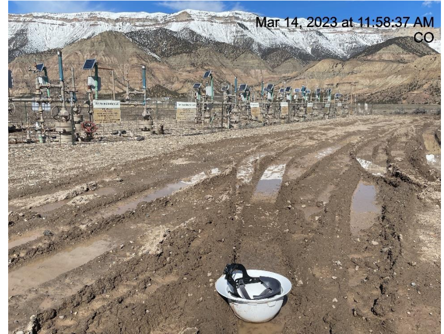
Photo # 2353 Lack of stabilization
