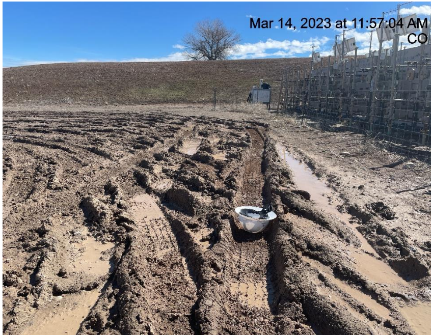
Photo # 2350 Lack of stabilization
