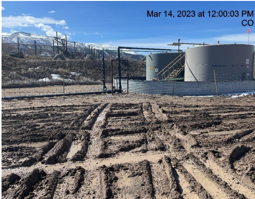
Photo # 2354 Lack of stabilization
