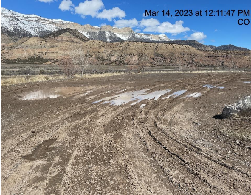
Photo # 2358 Lack of stabilization/Tracking onto lease road
