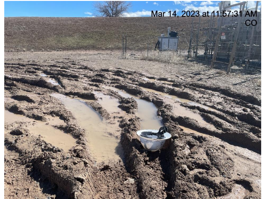
Photo # 2351 Lack of stabilization
