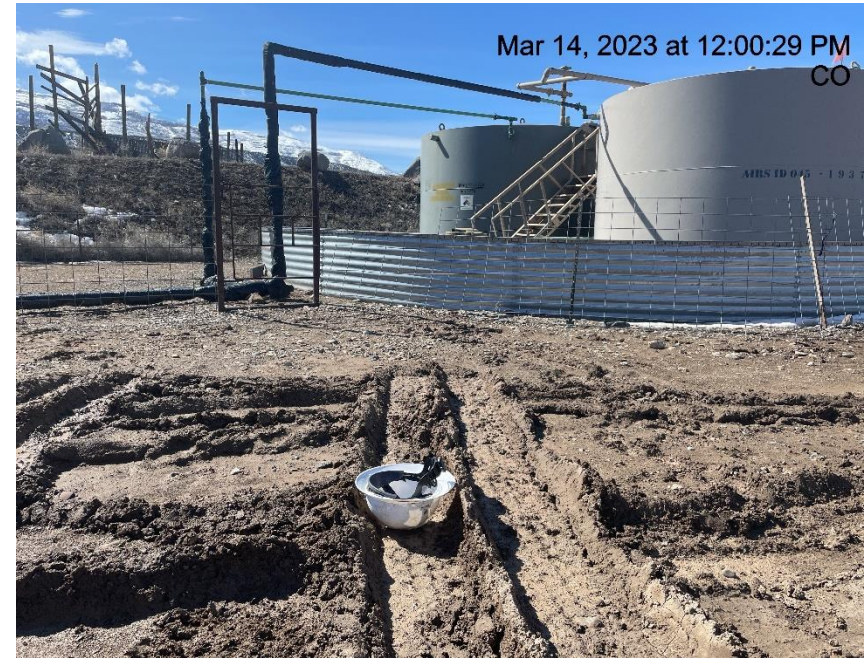
Photo # 2355 Lack of stabilization
