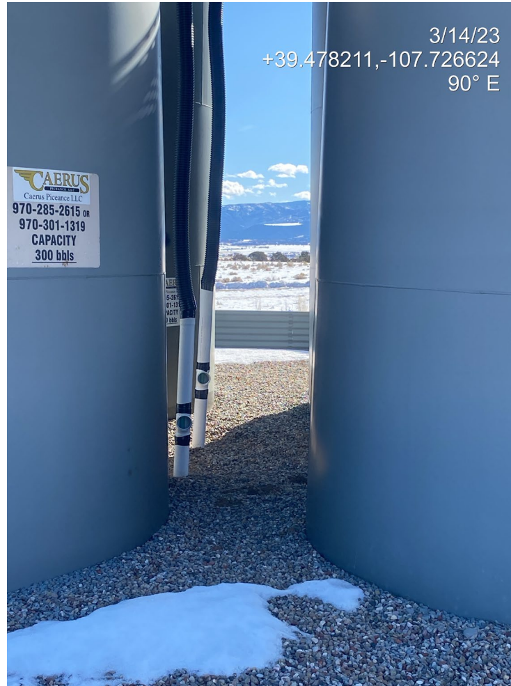
Photo 2. Photo shows open pipes at the tank battery lack wildlife protection BMPs.
