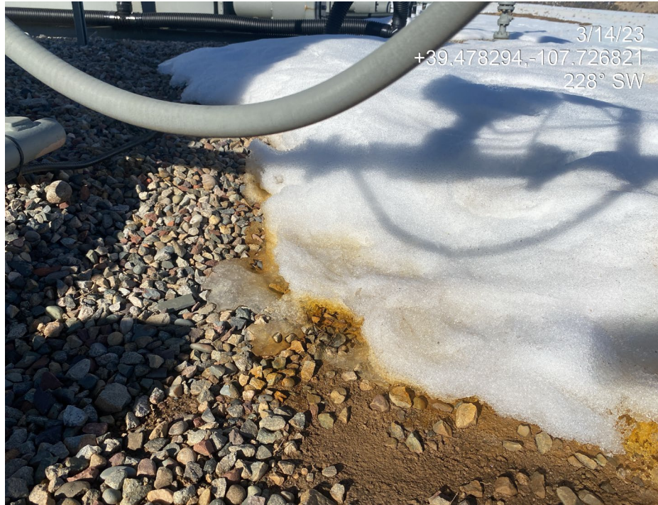
Photo 4. Photos show staining behind the separator for well API #045-07462.
