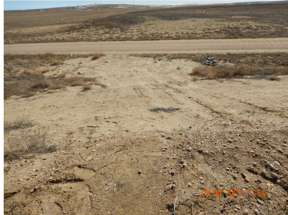
Photo 10. Photo taken from the northeastern location, facing South. Photo illustrates sediment has accumulated in the ditch/rip rap BMP.
