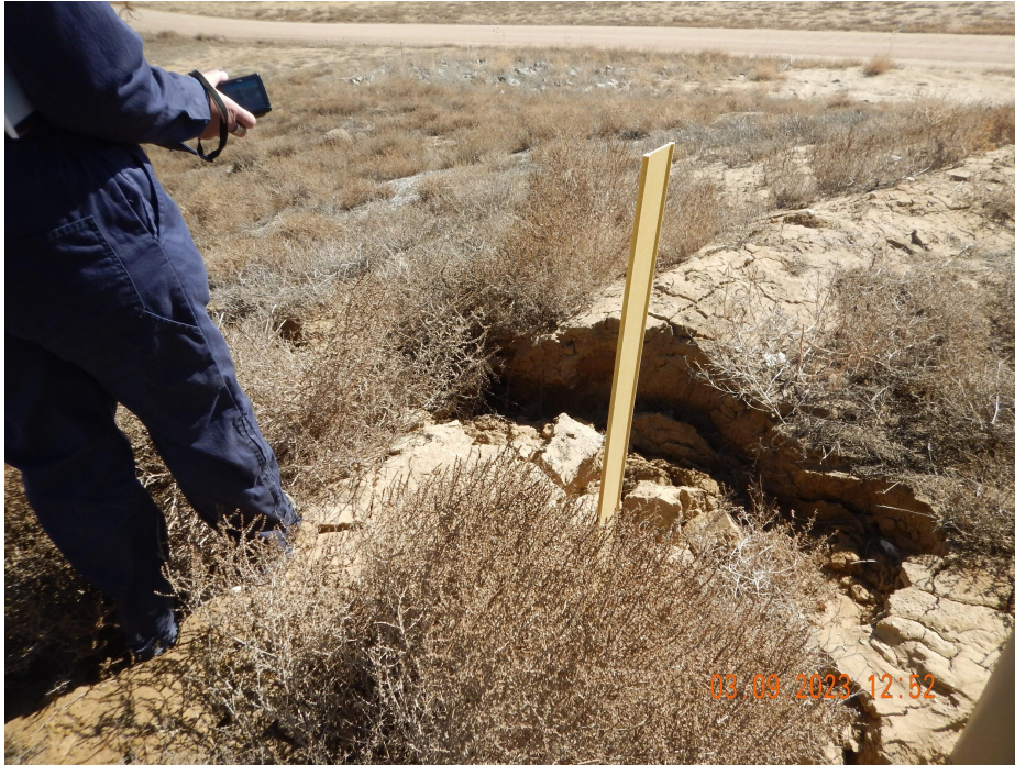
Photo 9. Photo taken from the northeastern location, facing East. Photo illustrates gully erosion along the ditch and berm BMP and weed establishment.
