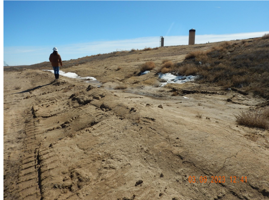
Photo 6. Photo taken from the northern location, facing East. Photo illustrates what appears to be a fill slope failure resulting in sediment discharge off location. See Photo 7.
