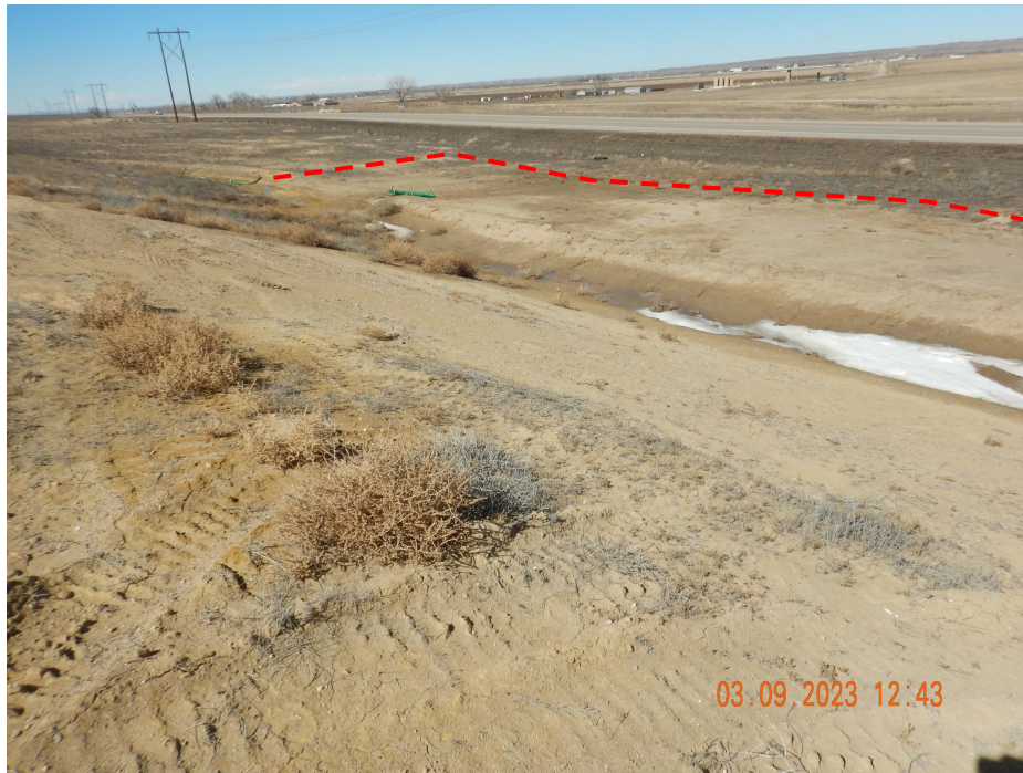
Photo 7. Photo taken from the northern location, on top of the fill slope, facing Northwest. Photo illustrates sediment discharge beyond the ditch BMP.
