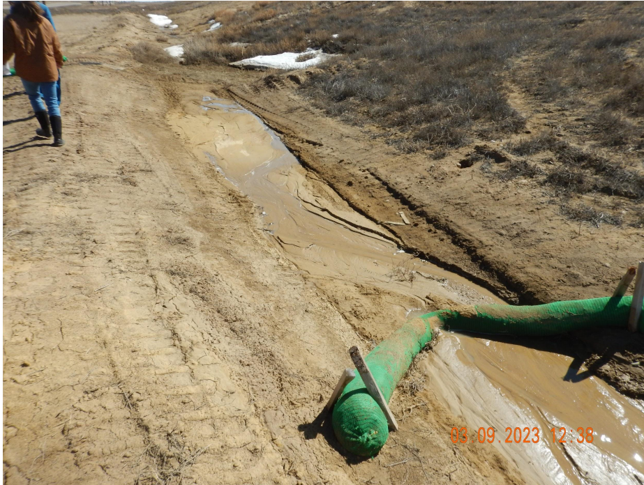
Photo 5. Photo taken from the northern location, facing East. Photo illustrates BMPs have not been maintained.
