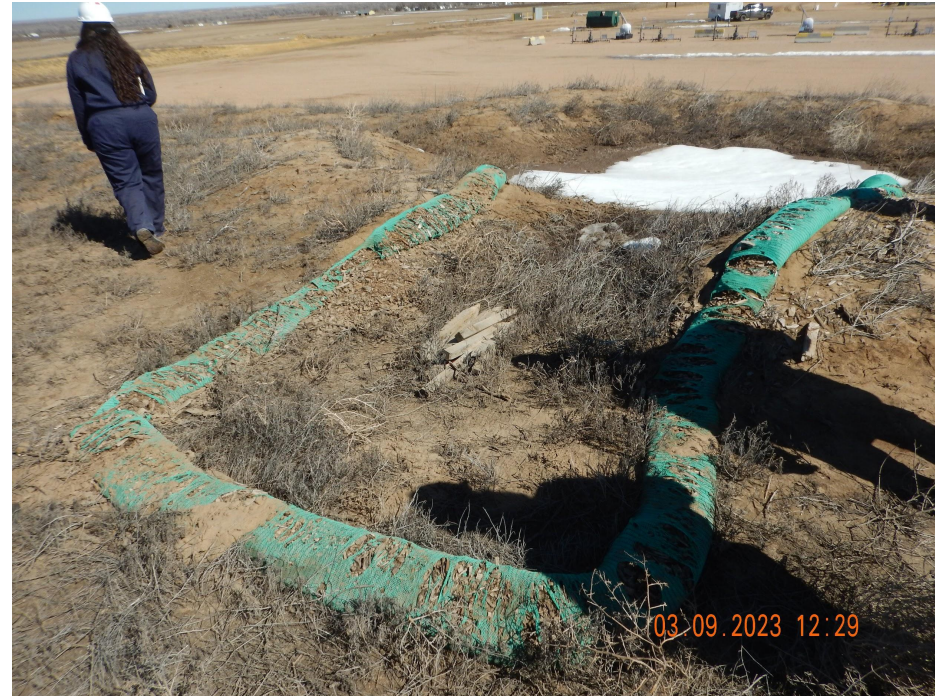
Photo 4. Photo taken from the western location, facing Northeast. Photo illustrates BMPs have not been maintained.
