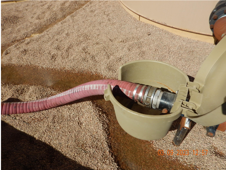
Photo 11. Photo taken from the produced water load out within secondary containment. Photo illustrates the hose has been left connected and is a potential safety concern with regards to a potential spill.
