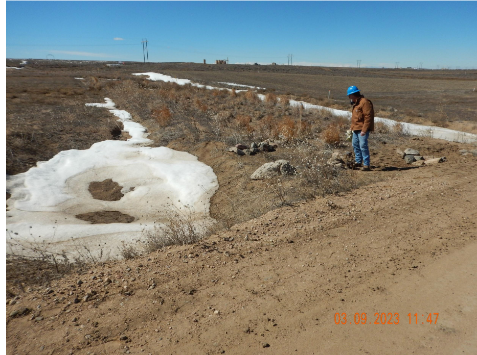
Photo 8. Photo taken from the western location, facing West. Photo illustrates concrete waste within rip rap of the culvert.
