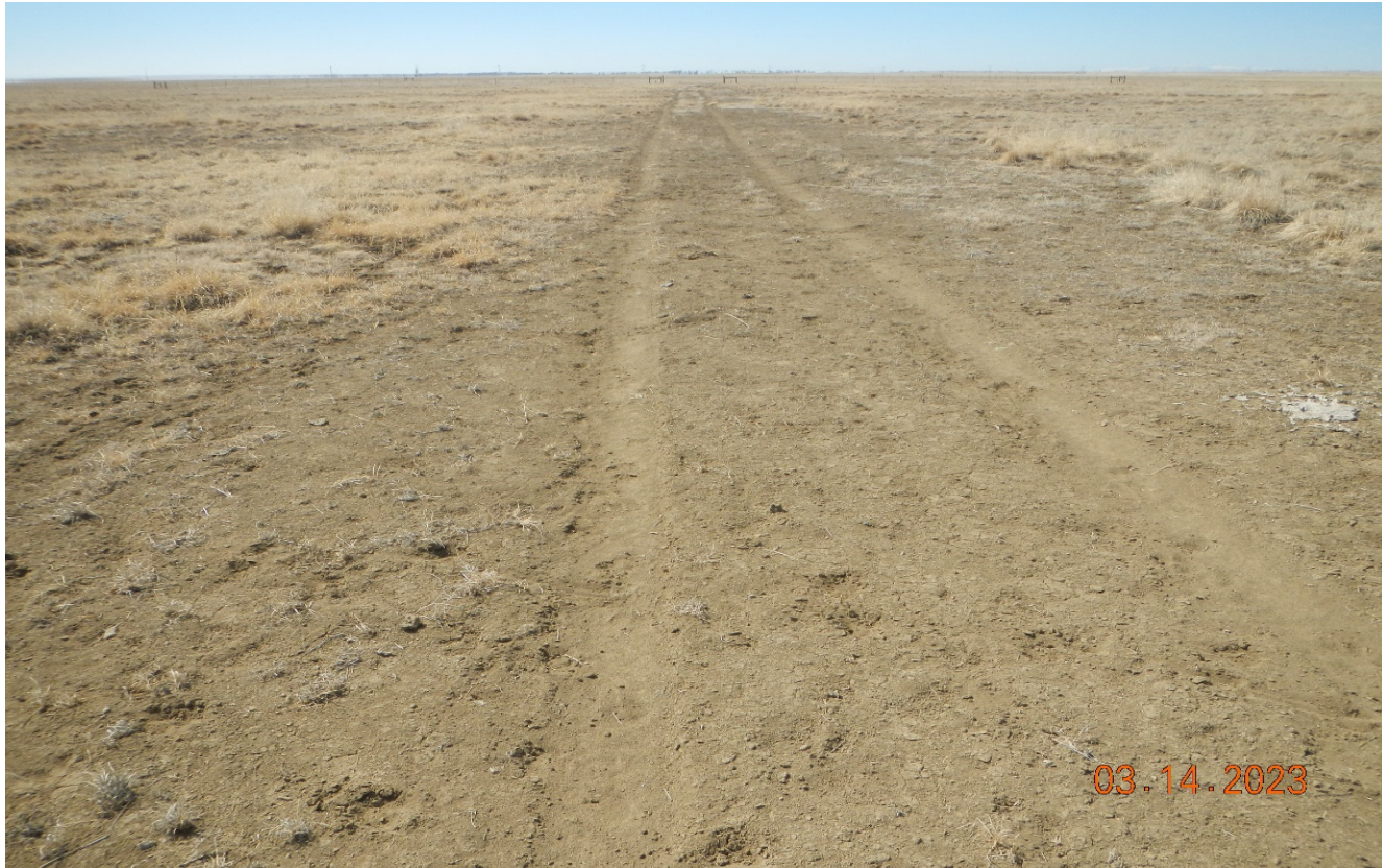
Photo 5. Facing southwest along the access road. The access road is bare of vegetation and needs to be reseeded.
