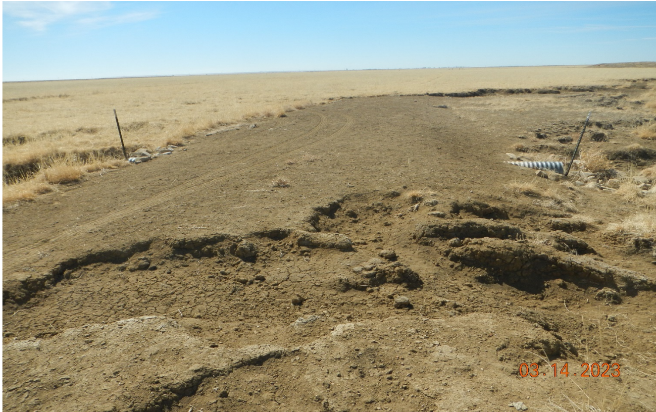
Photo 1. Facing southwest at Lat/Long:38.34638,-103.63420. This area has eroded and culvert is not functioning properly and should be removed or repaired..
