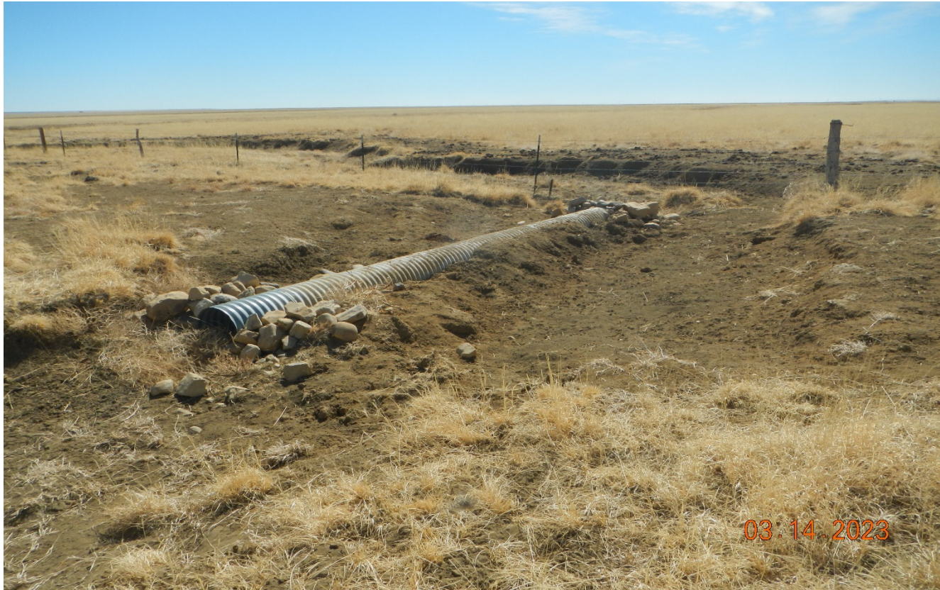
Photo 4. Facing southeast at Lat/Long:38.34370,-103.638545. This culvert has completely washed out and should be removed or repaired. A dry crossing may be more appropriate at this area due to frequent flooding.
