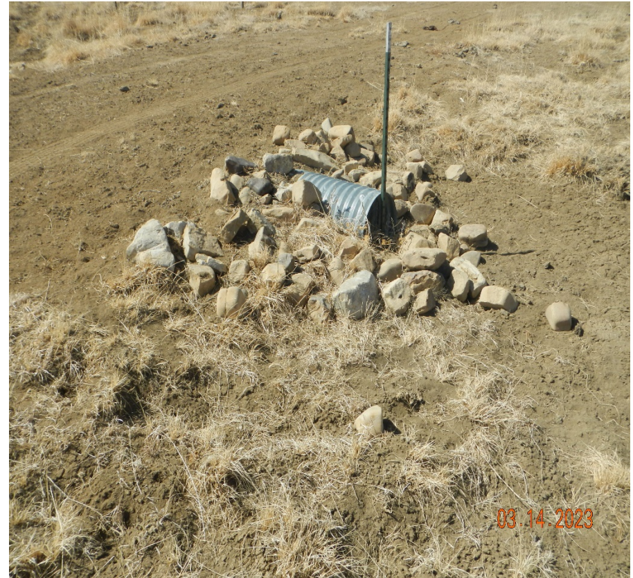
Photo 3. There are rocks piled up in front of the culvert which will impede water flow.
