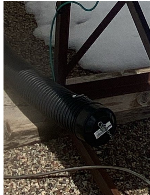
Photo 1. Photos show a cap has been installed on piping at the tank battery.
