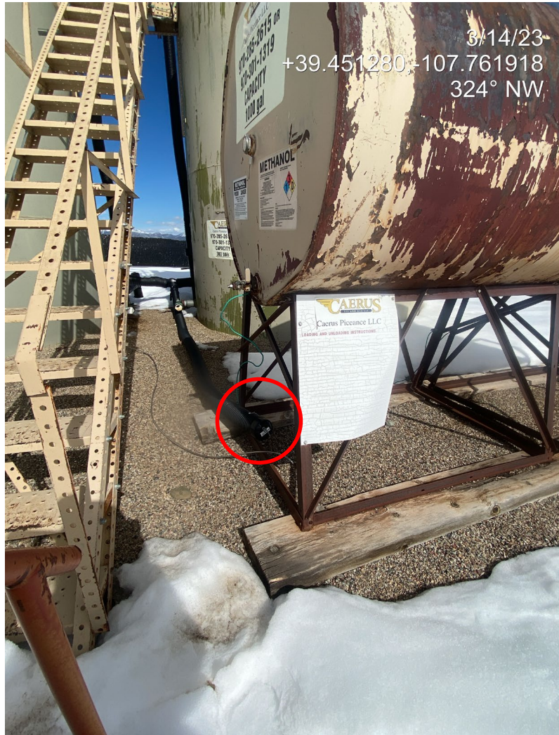
Photo 1. Photos show a cap has been installed on piping at the tank battery.
