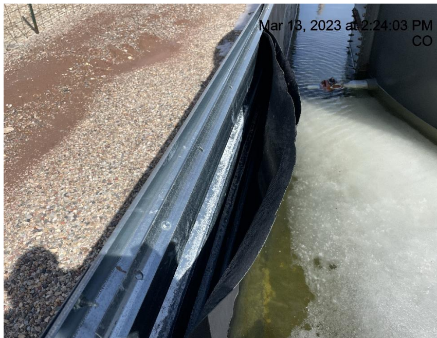
Photo # 2312 Containment needs maintenance
