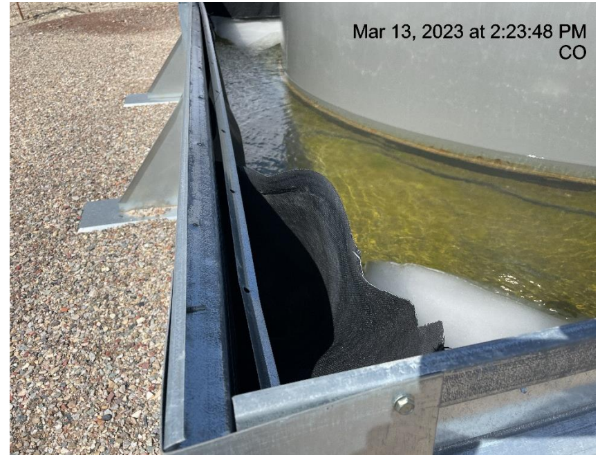
Photo # 2311 Containment needs maintenance
