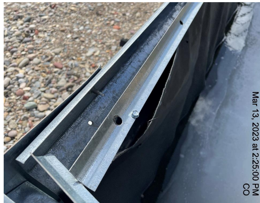
Photo # 2313 Containment needs maintenance
