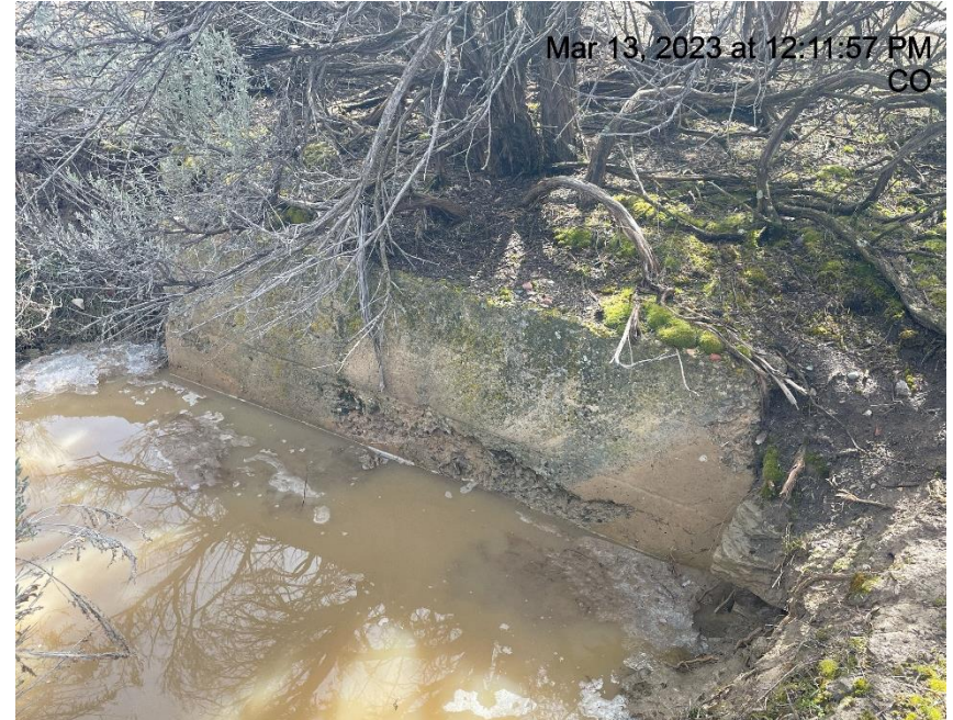
Photo # 2227 Culvert needs maintenance – Culvert on access road, 180 ft east of RWF 22-29 pad
