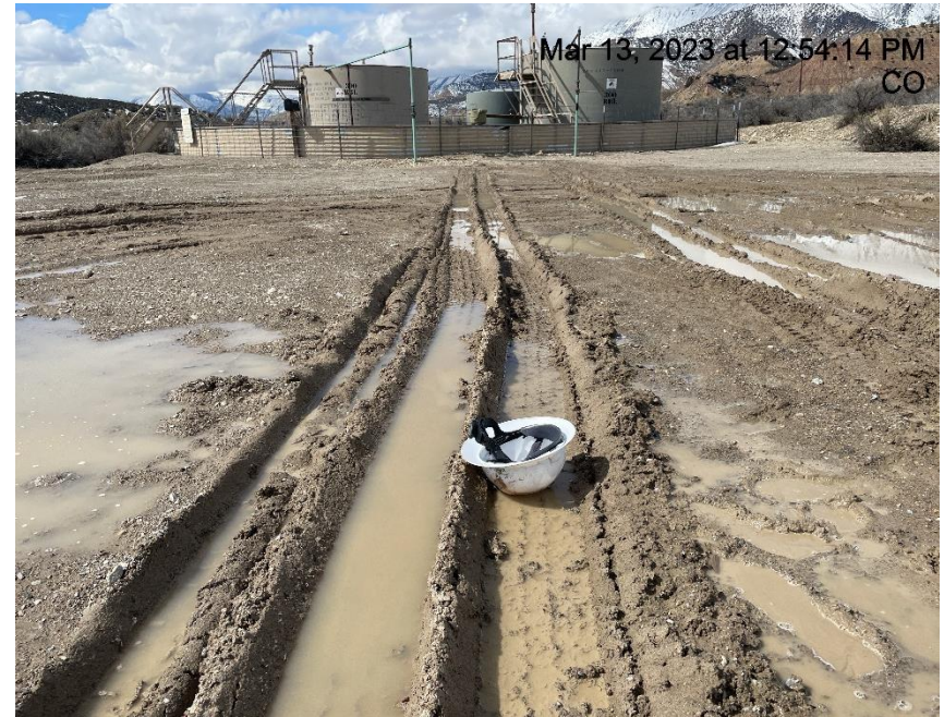
Photo # 2248 Lack of stabilization
