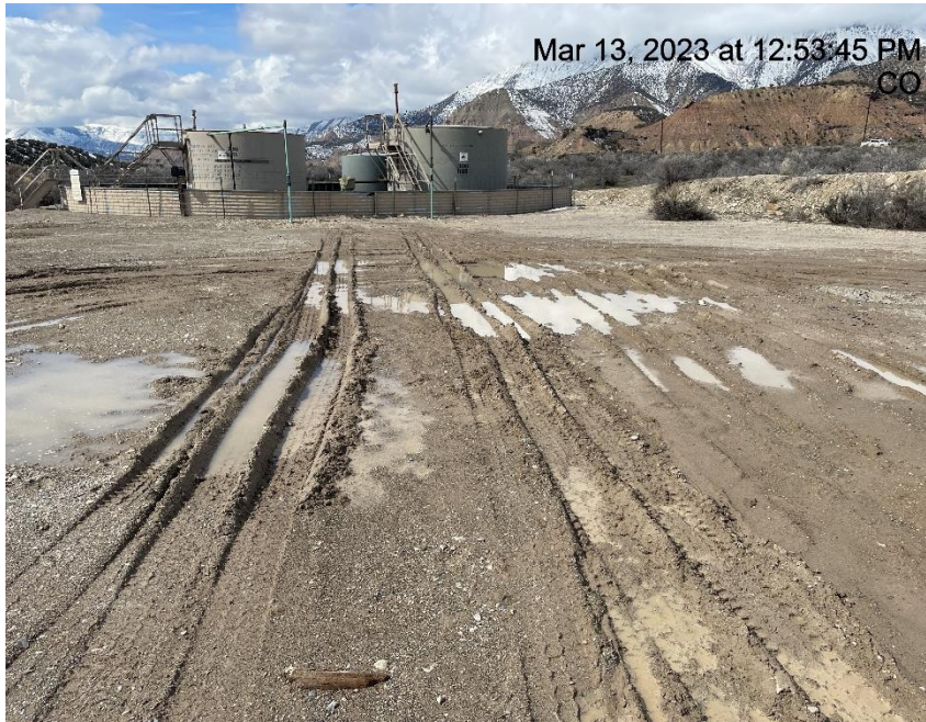
Photo # 2246 Lack of stabilization
