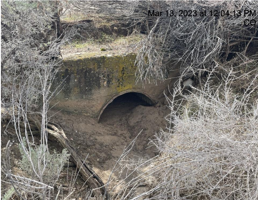
Photo # 2226 Culvert needs maintenance – Culvert on access road, 40 ft east of RWF 22-29 pad
