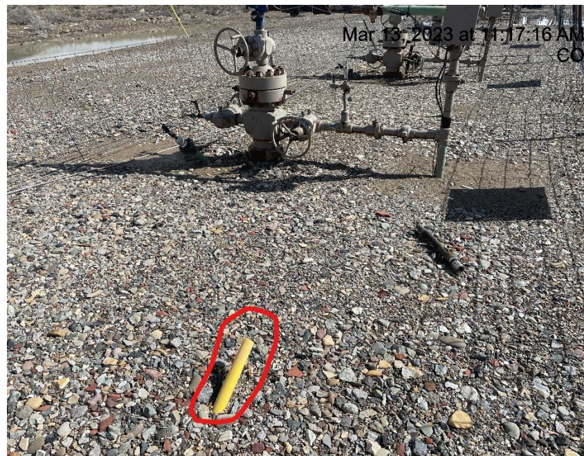
Photo # 2213 Improperly marked deadman
