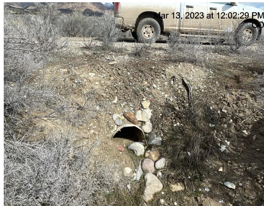
Photo # 2223 Culvert needs maintenance – 160 ft west of location on spur road
