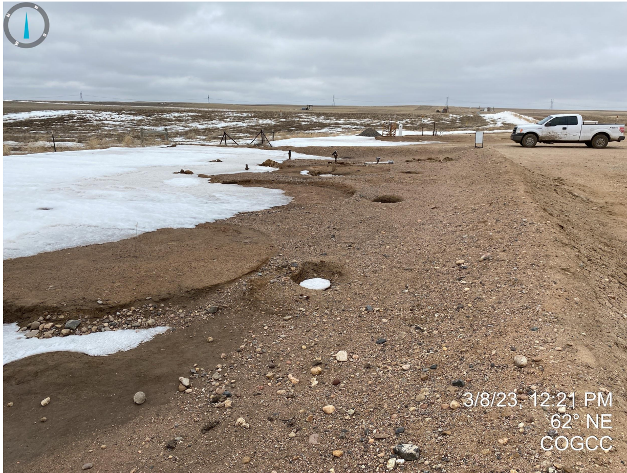
Photo 1. Facing northeast from the former tank battery. Photo illustrates that tanks and other equipment have been removed, however, unmarked risers and piping were still in place and need to be removed.
