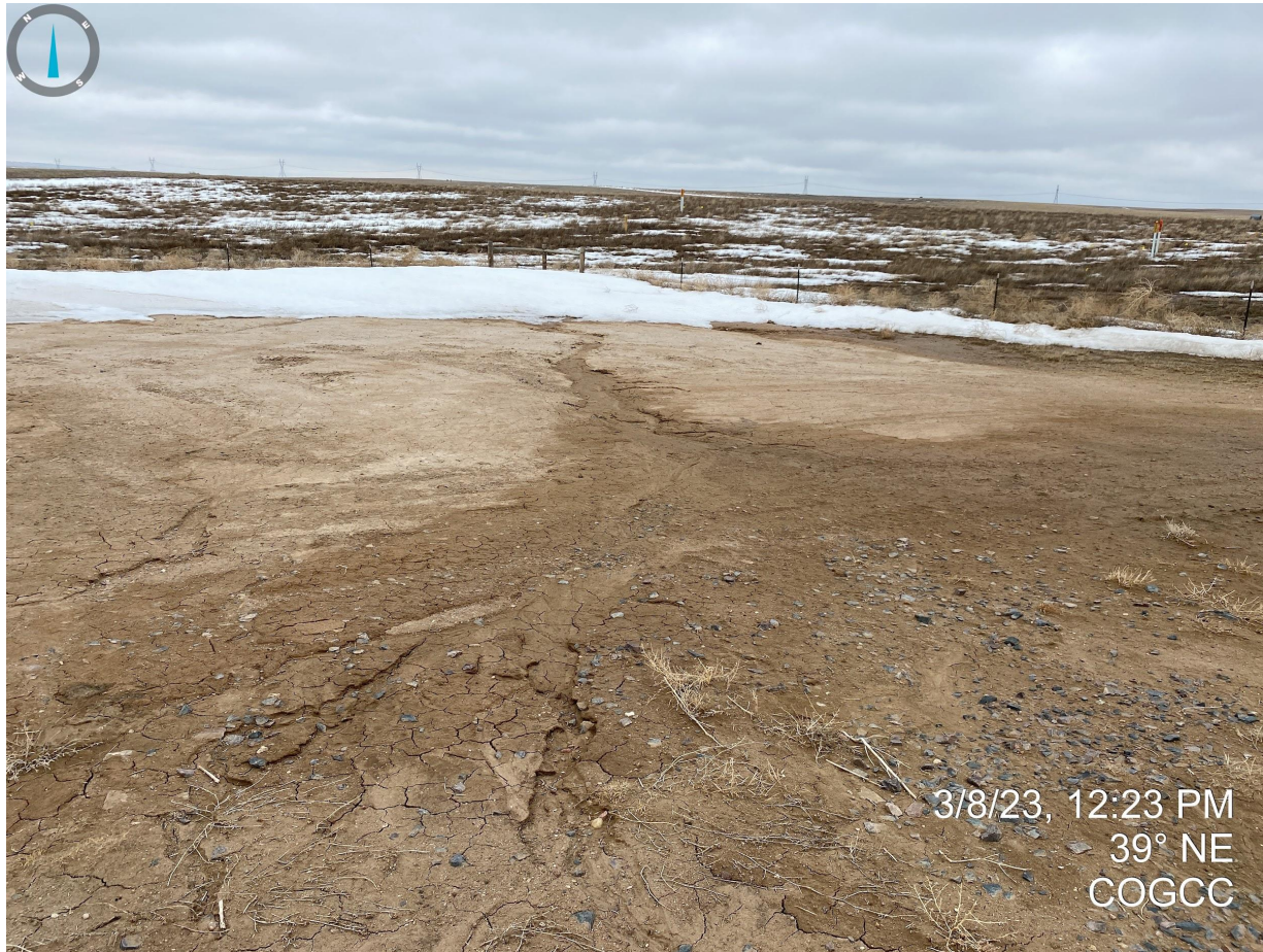
Photo 4. Facing northeast from the location, near the former pit location. Rill erosion was occurring on the pad surface and appeared to be moving off location. Snow cover prevented full observation of the stormwater travel and any BMPs that may or may not be in place to prevent stormwater from exiting off location. The working pad will need to be stabilized to prevent further erosion.
