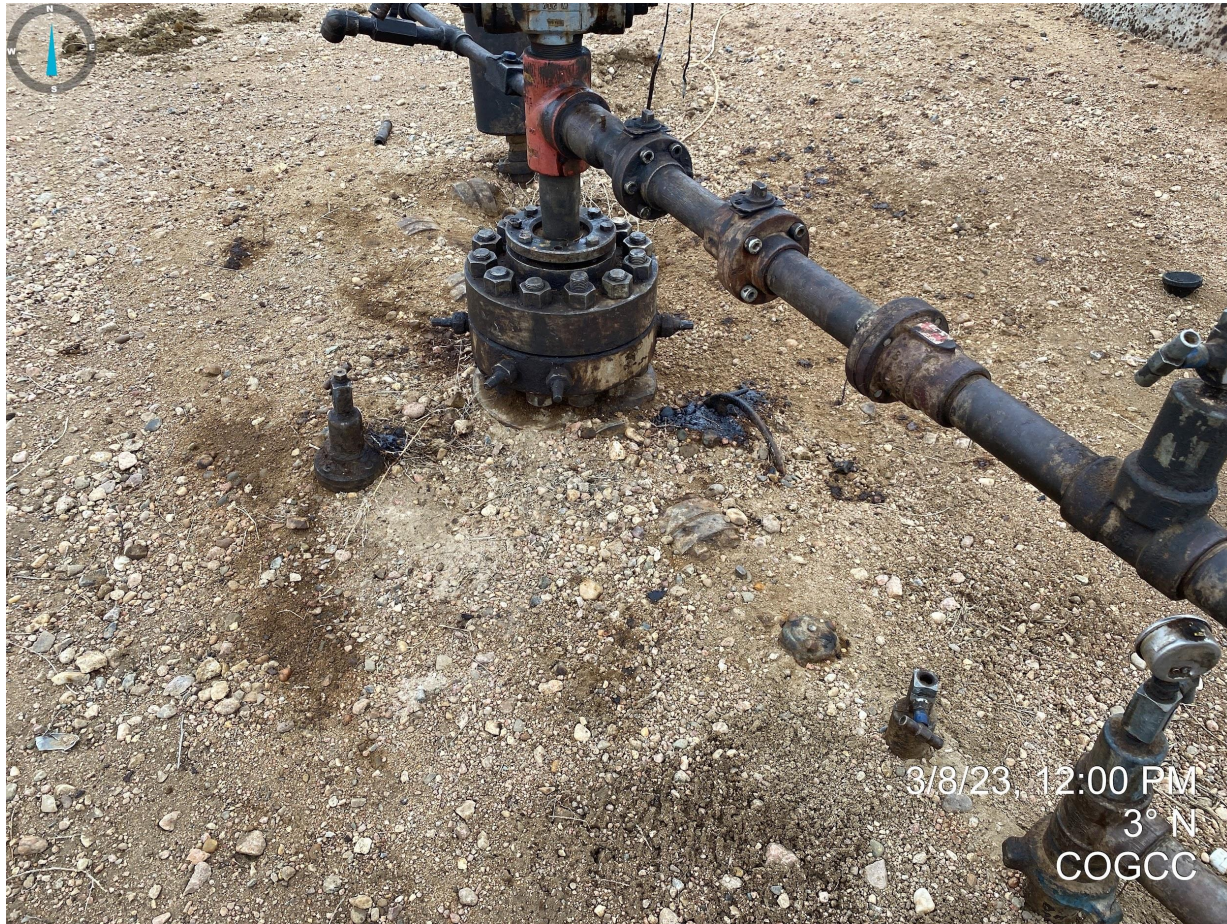
Photo 3. Oily waste/stained soil near wellhead.
