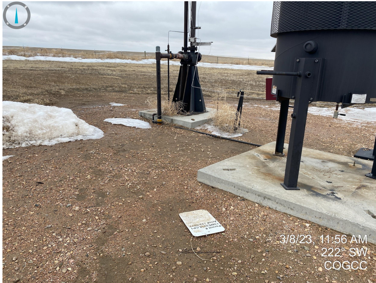
Photo 1. Facing southwest at flare and combustor. Tumbleweed accumulations were observed in and around equipment and are now considered debris as they present a fire hazard.
