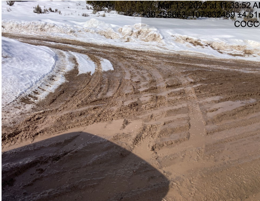
Location entrance lacks tracking BMP's
