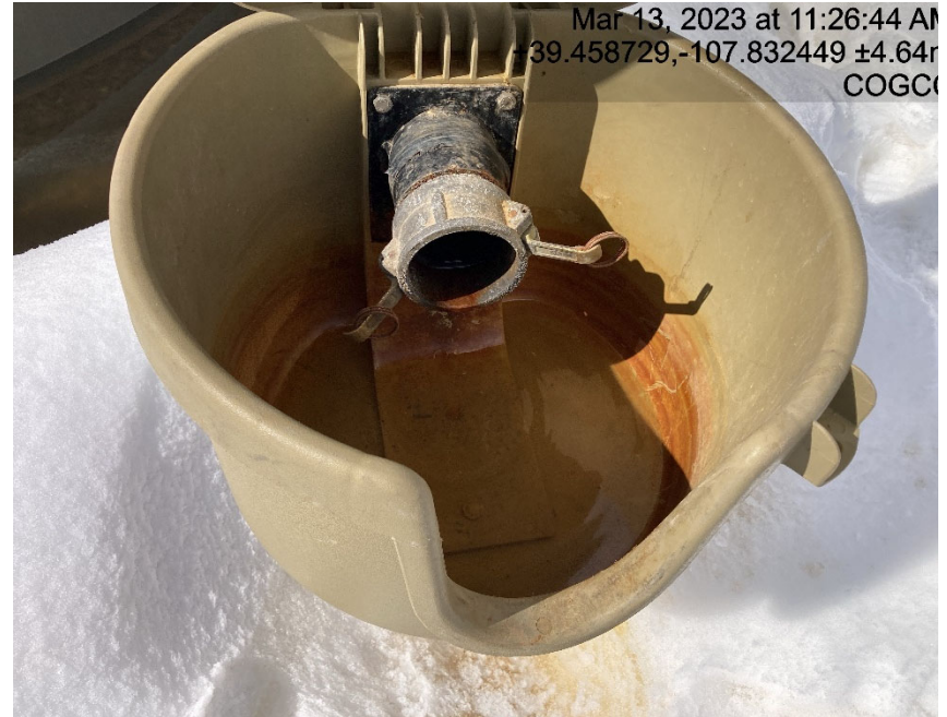
Line from tank missing cap/plug
