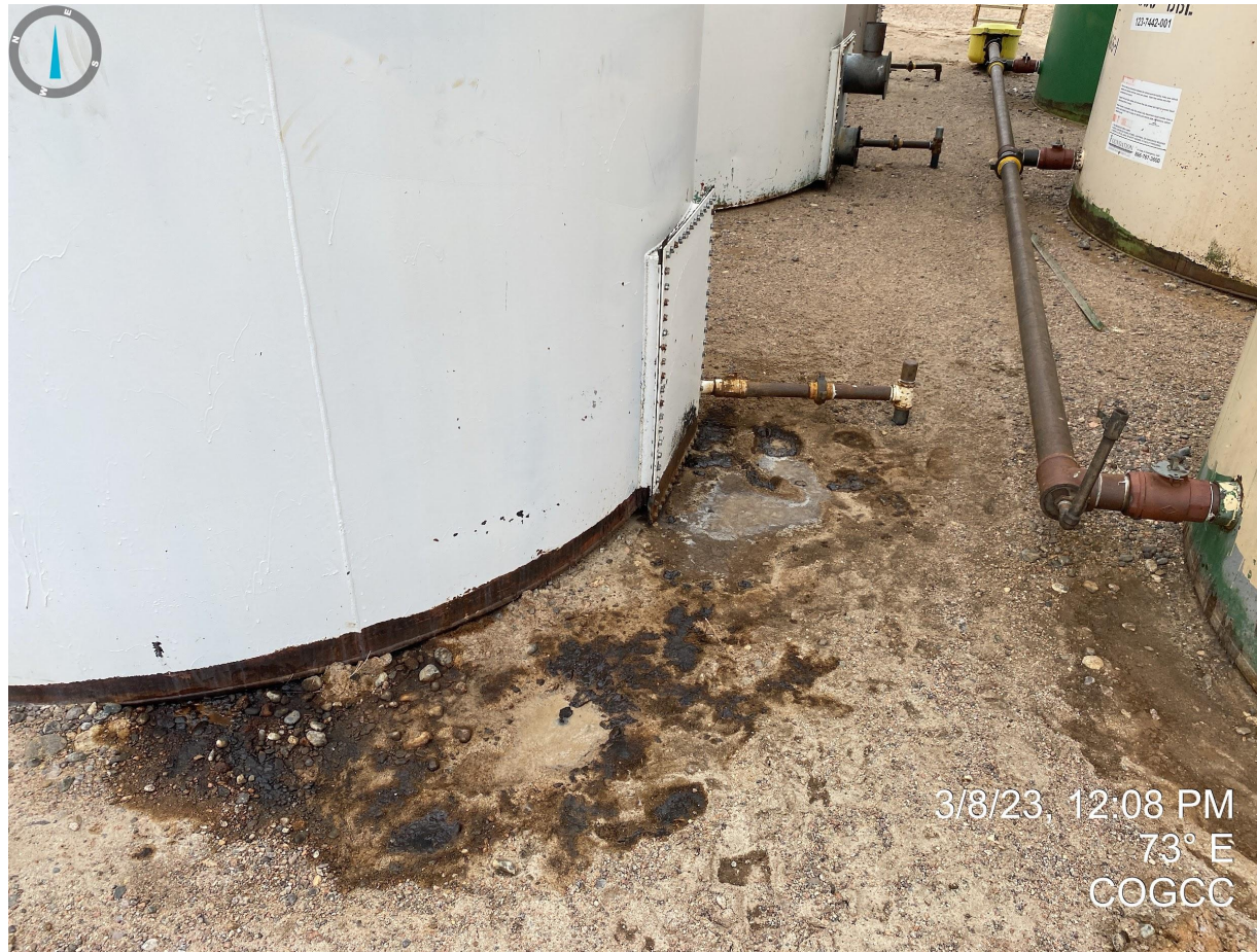
Photo 1. Facing east at the northwest-most tank battery. Unknown fluid observed around bottom of tank. The tank itself will need to be inspected per Rule 609.b and the stained soil will need to be disposed of per Rule 905.e.
