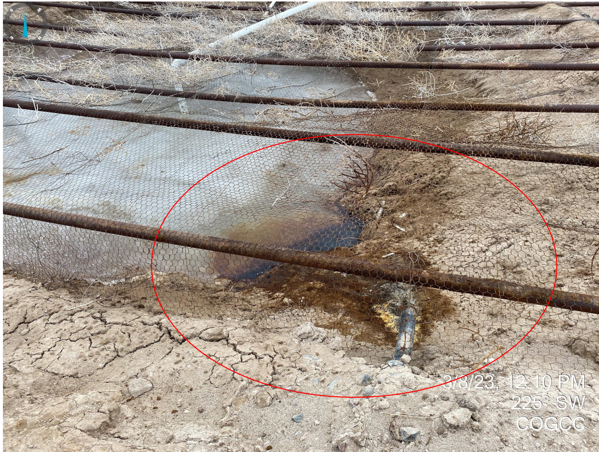
Photo 3. Facing southwest at pit. Hydrocarbons observed within the pit will need to be properly cleaned up and disposed of per Rule 909.d.
