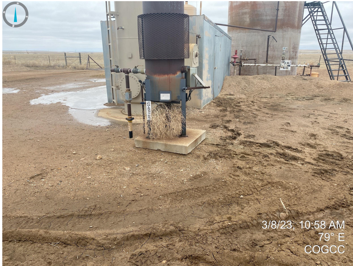
Photo 1. Facing east towards production area. Tumbleweed accumulations were observed in and around equipment and need to be removed as they present a fire hazard.
