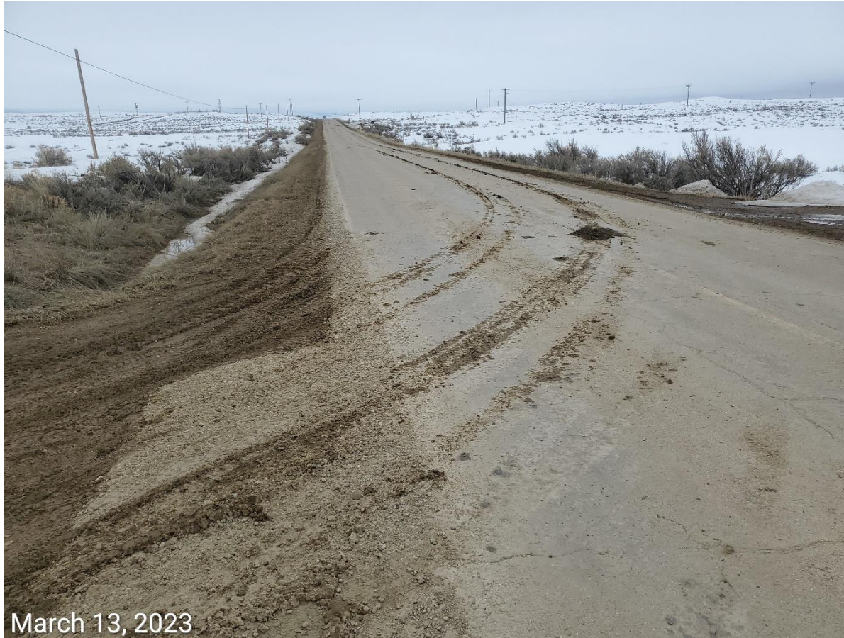
Photo 5: See comments under photo 1. Photo also shows tracking from access road onto Hwy 64.
