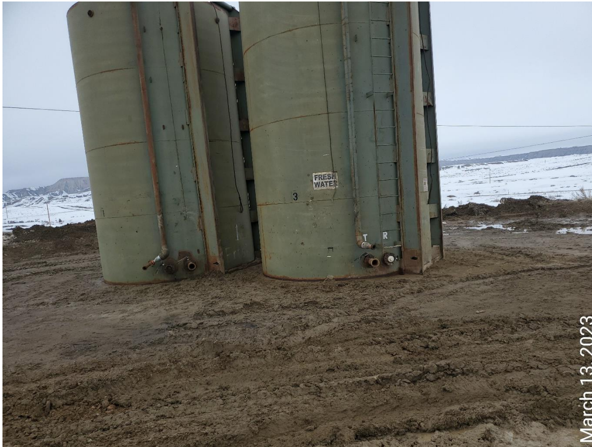
Photo 19: Photo shows tank on Location missing required labeling.
