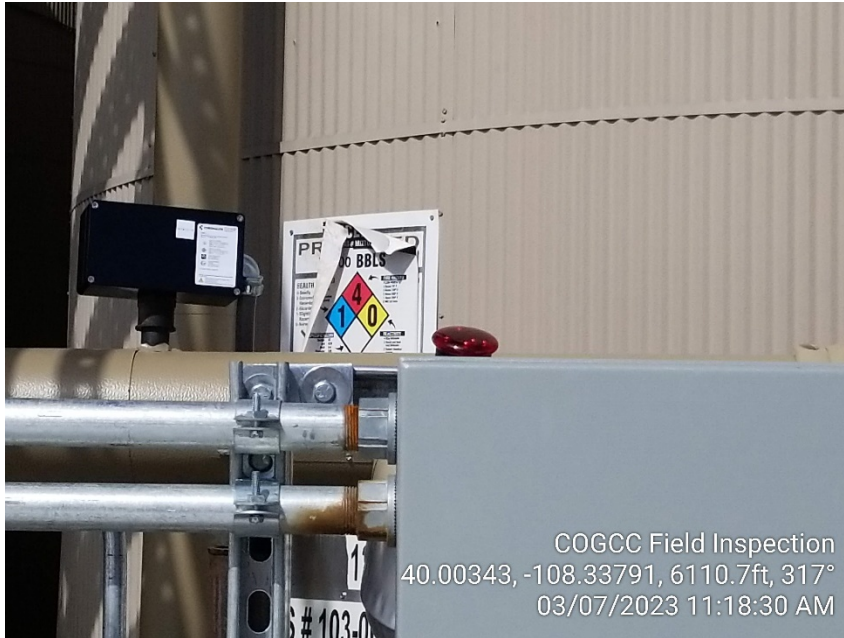
Photo #9 – Volume labels and NFPA placards on several tanks in need of repair.
