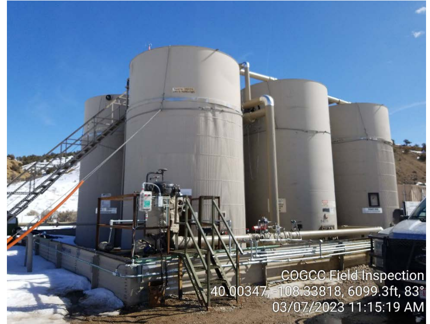
Photo #2 – View of tank battery from northwest. Note filter pot in northwest corner of tank battery.
