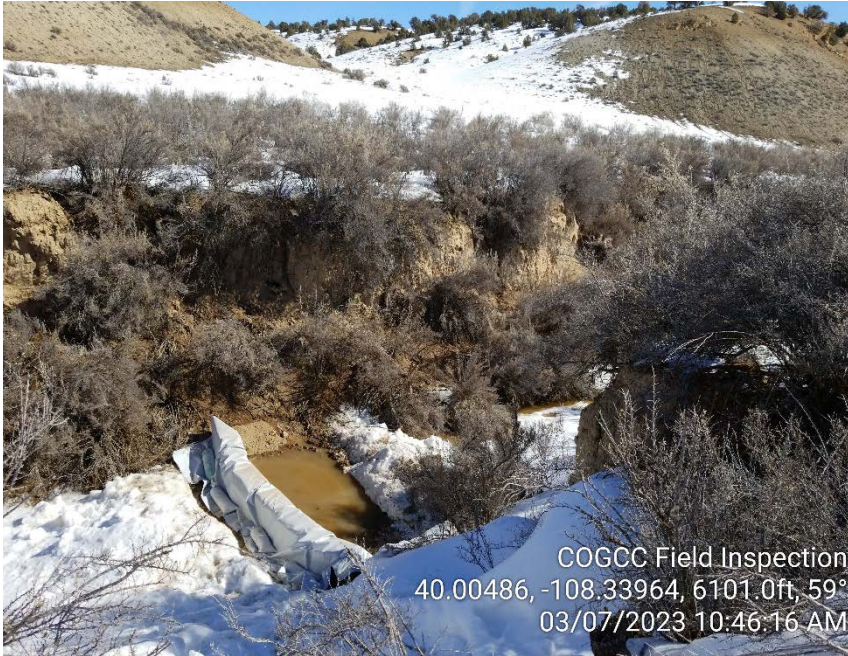
Photo #7 – Check dam inside of impacted intermittent drainage.
