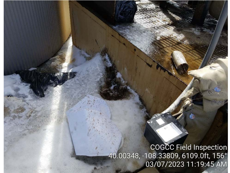
Photo #6 – A filter sock had fallen from its storage area into tank battery secondary containment on inspection date. Due to likelihood of high winds in the area, it is recommended that the Operator utilize a dedicated storage container to prevent loss of unused equipment.
