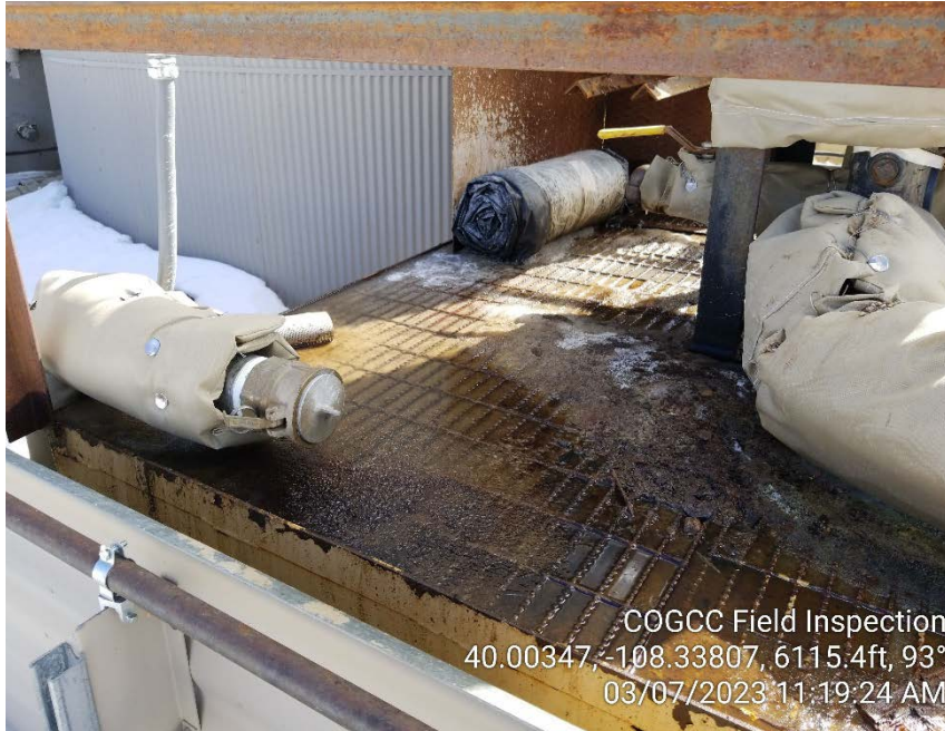
Photo #3 – Filter pot secondary containment device was filled with fluids (commingled hydrocarbons and snowmelt) during inspection.
