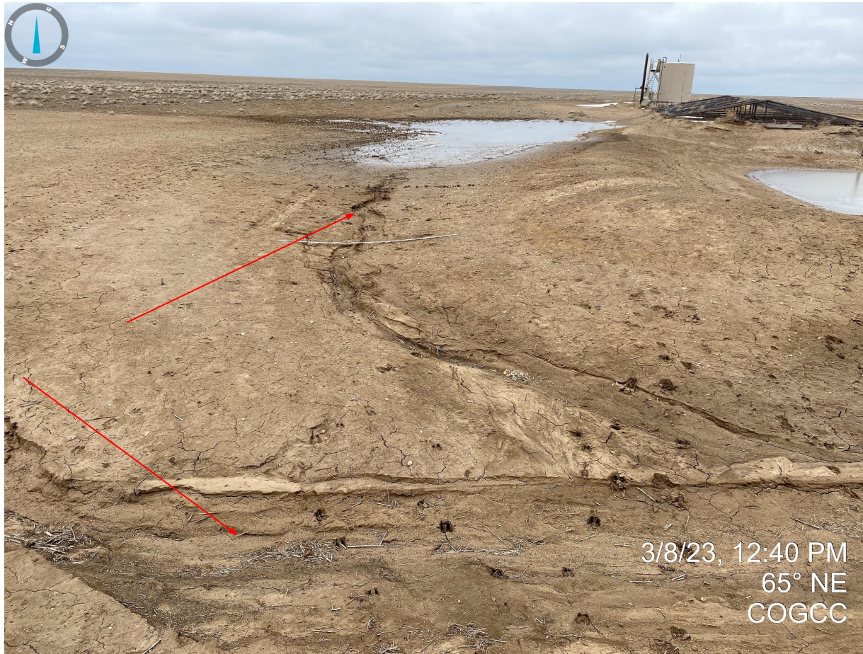
Photo 1. Facing northeast near pits. Photo illustrates rill and gully erosion occurring on location. No BMPs were observed on location to manage stormwater. Sediment laden stormwater was also observed to have migrated off location into adjacent lands (see Photos 5 & 6). Stormwater BMPs will need to be implemented immediately to prevent further off location degradation.
