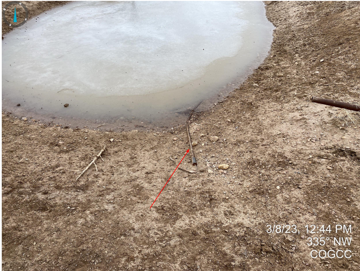
Photo 12. Facing northwest at pit. Sucker rod observed within pit is considered used equipment and needs to be removed.
