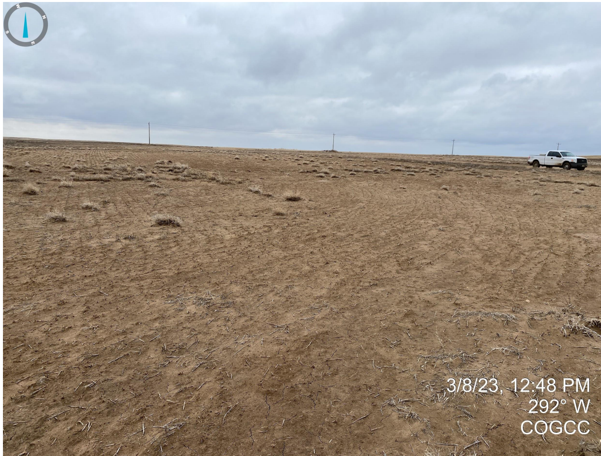
Photo 8. Facing west near reclaimed well location. It appears the operator has performed final reclamation activities with evidence of contouring and grading, and removal of debris and equipment.
