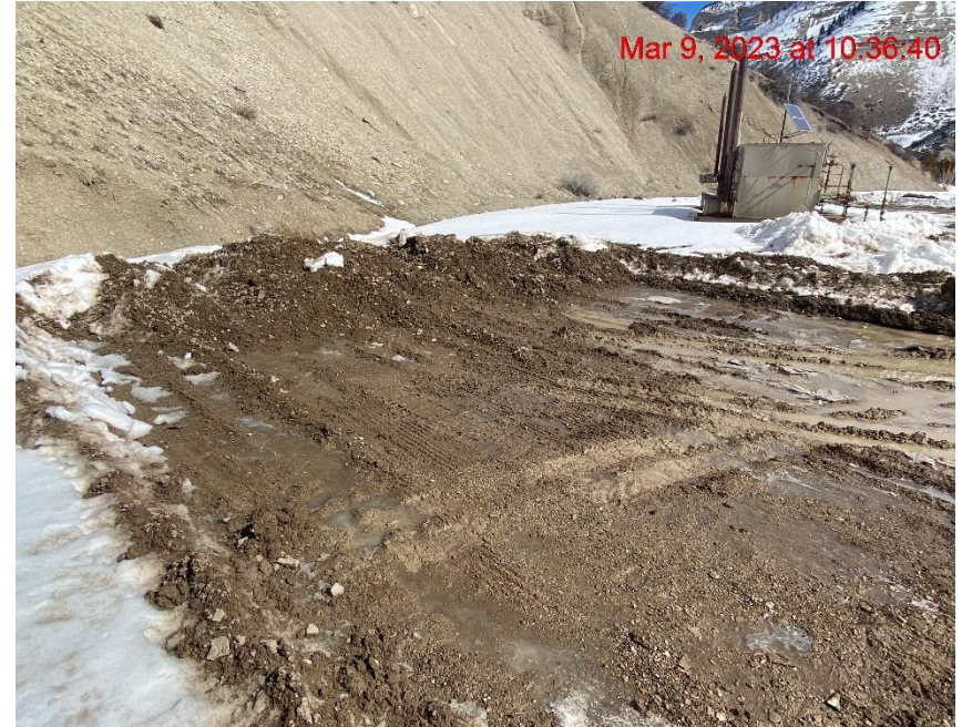
Lack of Stabilization/Soil Stockpile – Photo #01277
