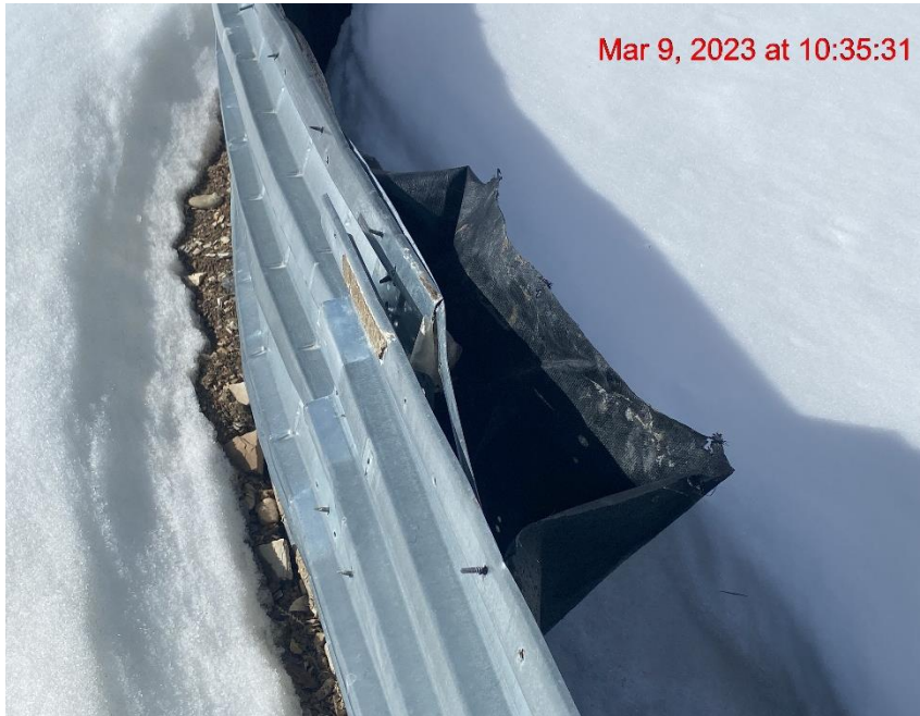
Berm Wall Damage – Photo #01274
