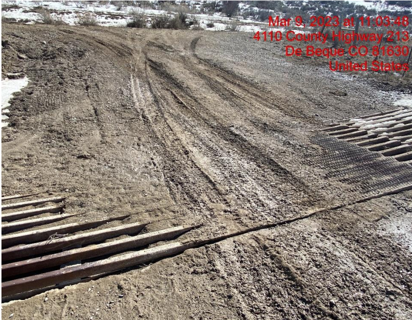
Inadequate Tracking BMP – Photo #01288
