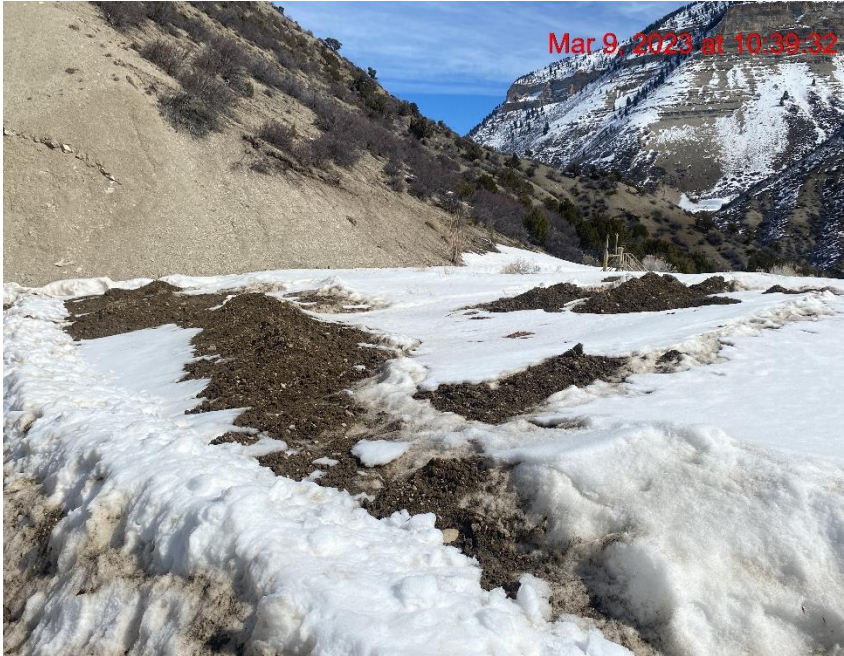
Unprotected Soil Stockpiles – Photo #01281
