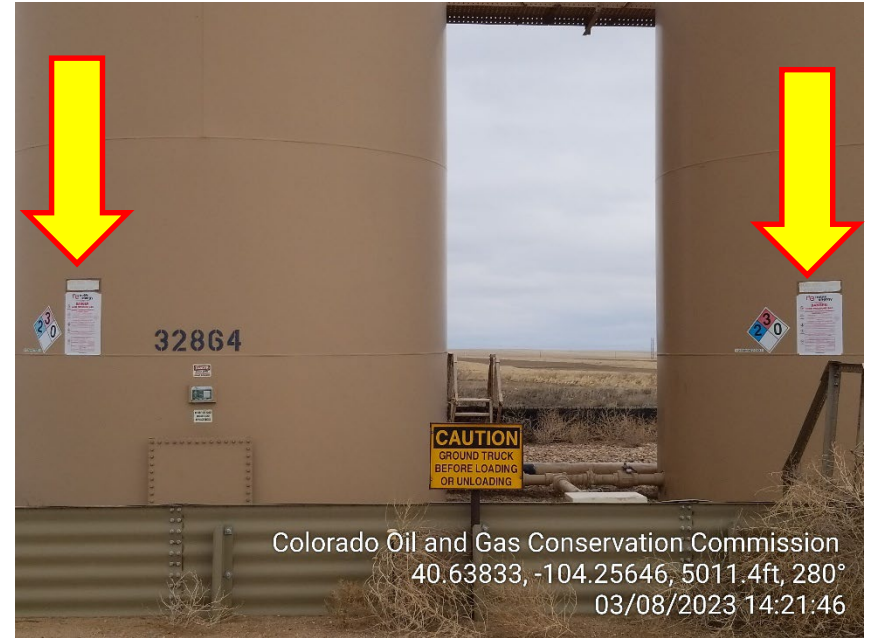
Photo 4 – Content and Capacity Labels
