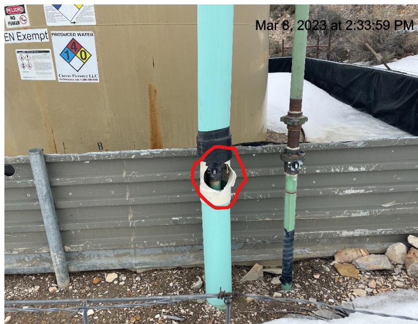
Photo # 2020 Flowline heating insulation open ended
