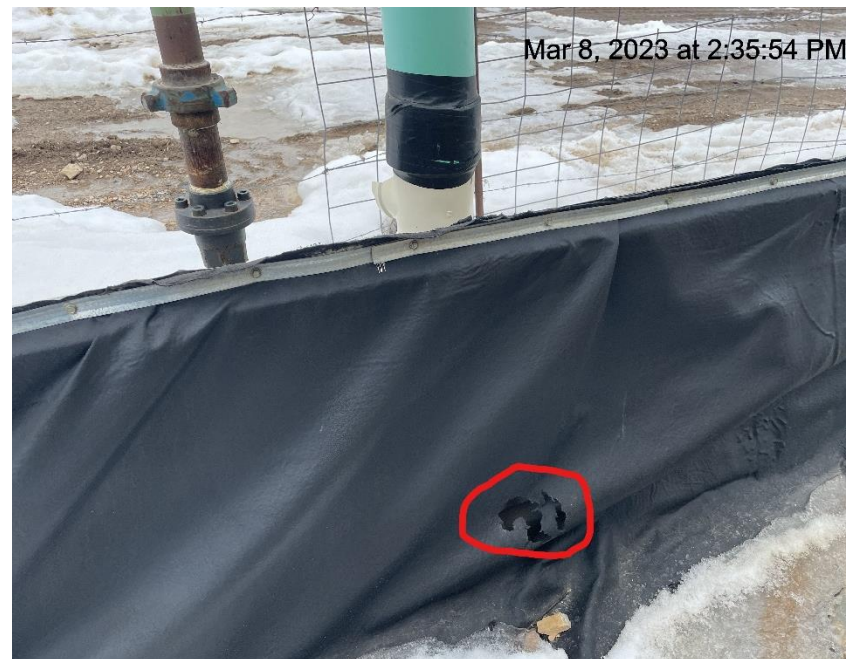
Photo # 2024 Containment needs maintenance
